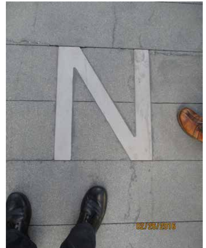
EMBEDDED METAL LETTERS ON PLATFORM
