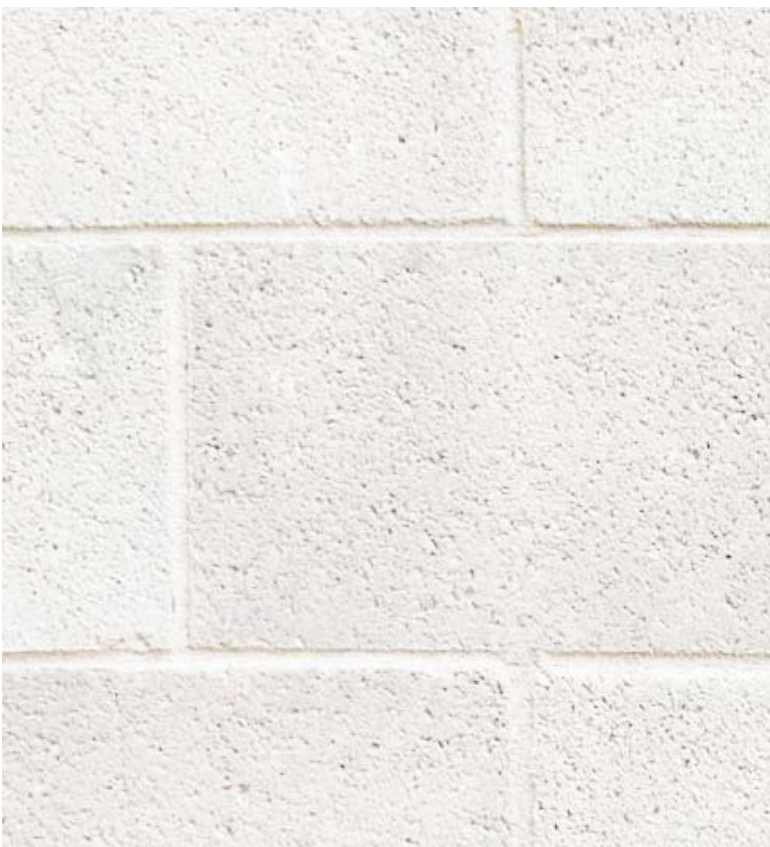
PAINTED C.M.U. BLOCK WALLS
