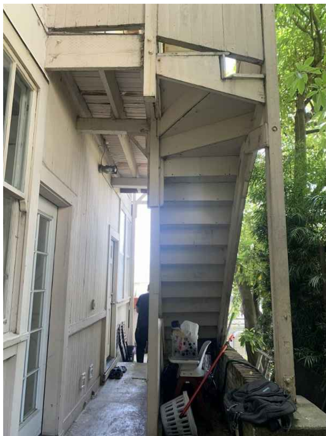
5 THE FIRST FLOOR STRINGERS, POSTS, AND FOOTINGS
