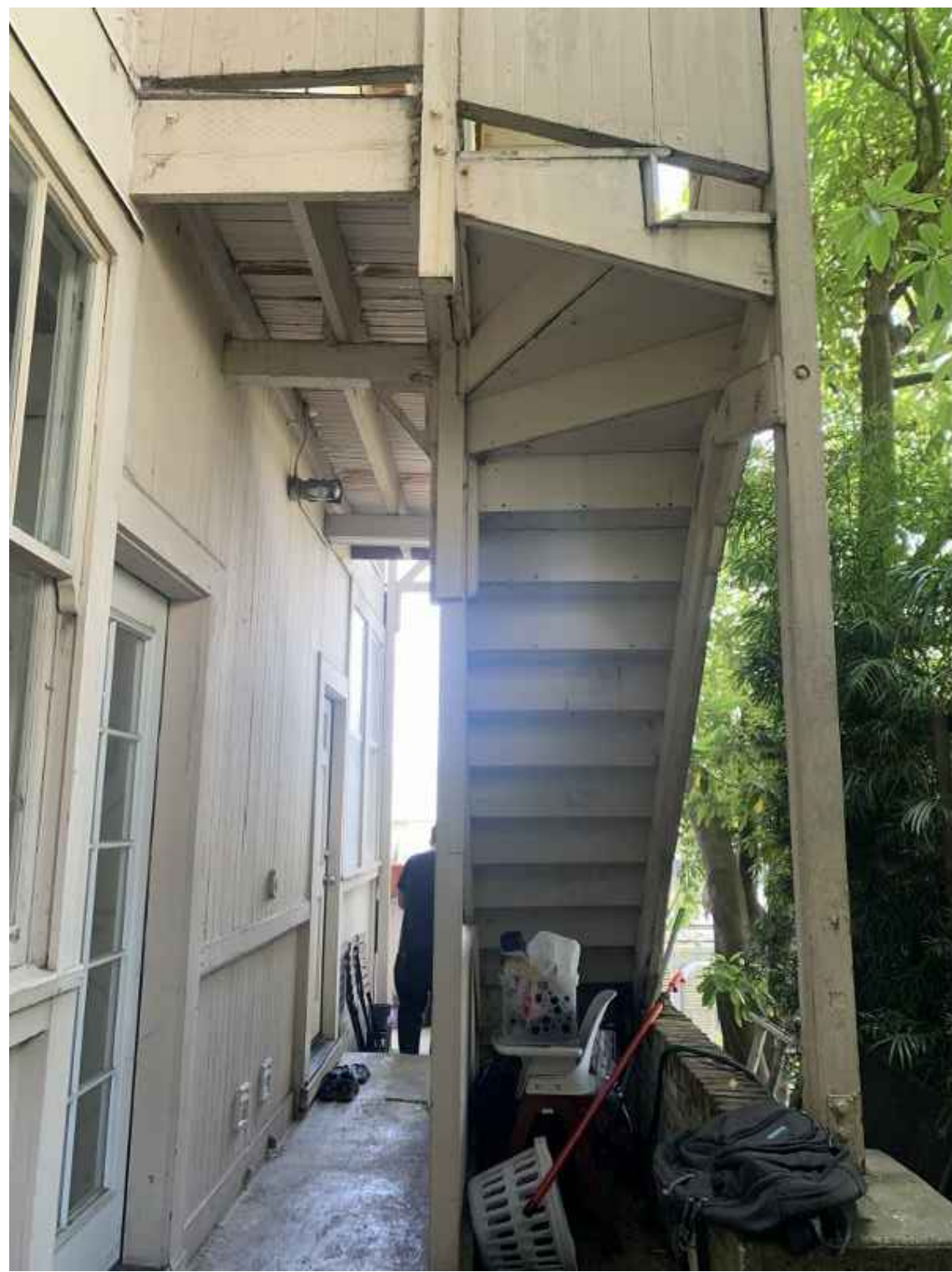
5 1ST FLOOR STRINGERS, POSTS, & FOOTINGS
