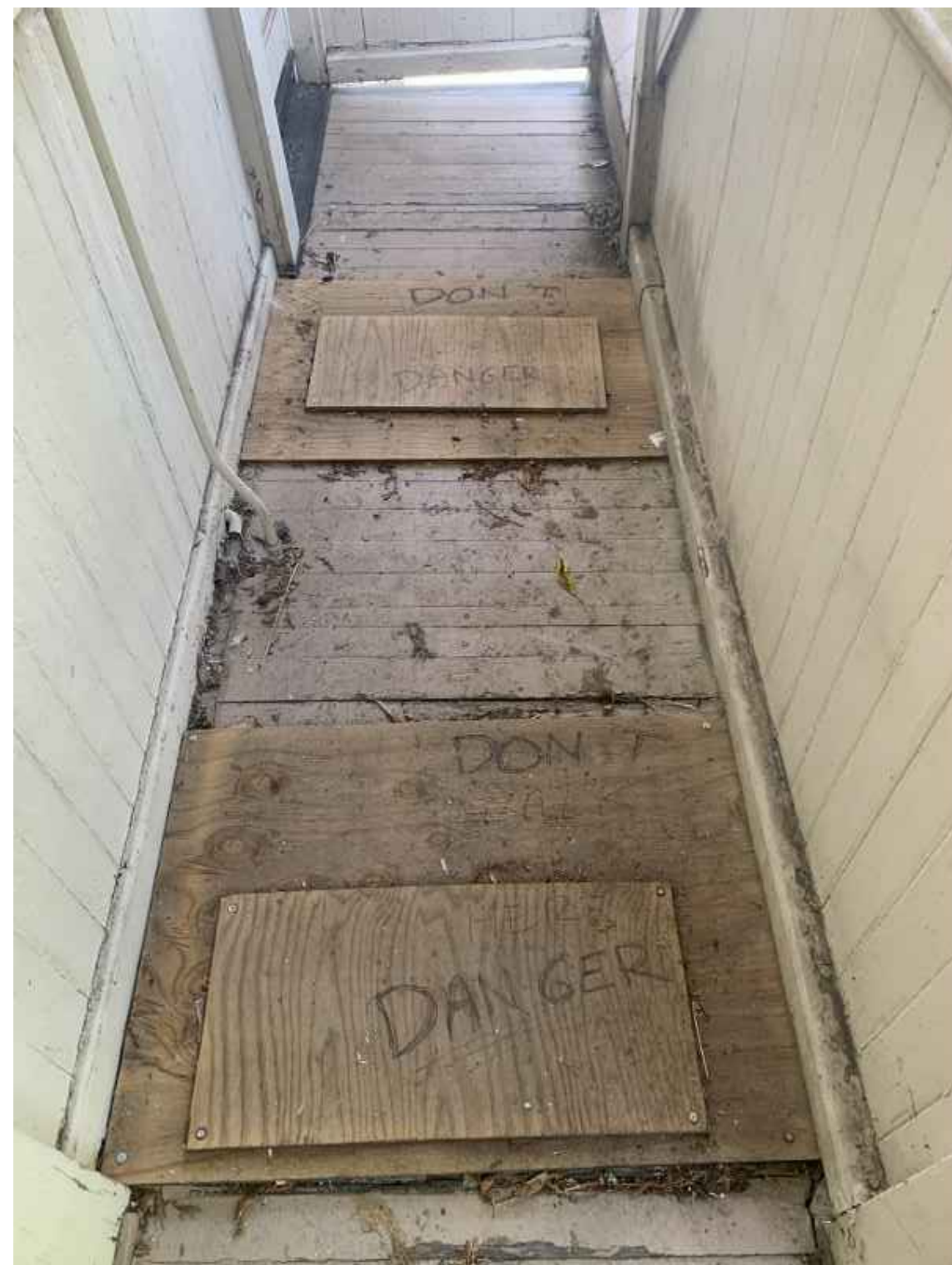
6 TYPICAL DAMAGED SLOPING LANDING
