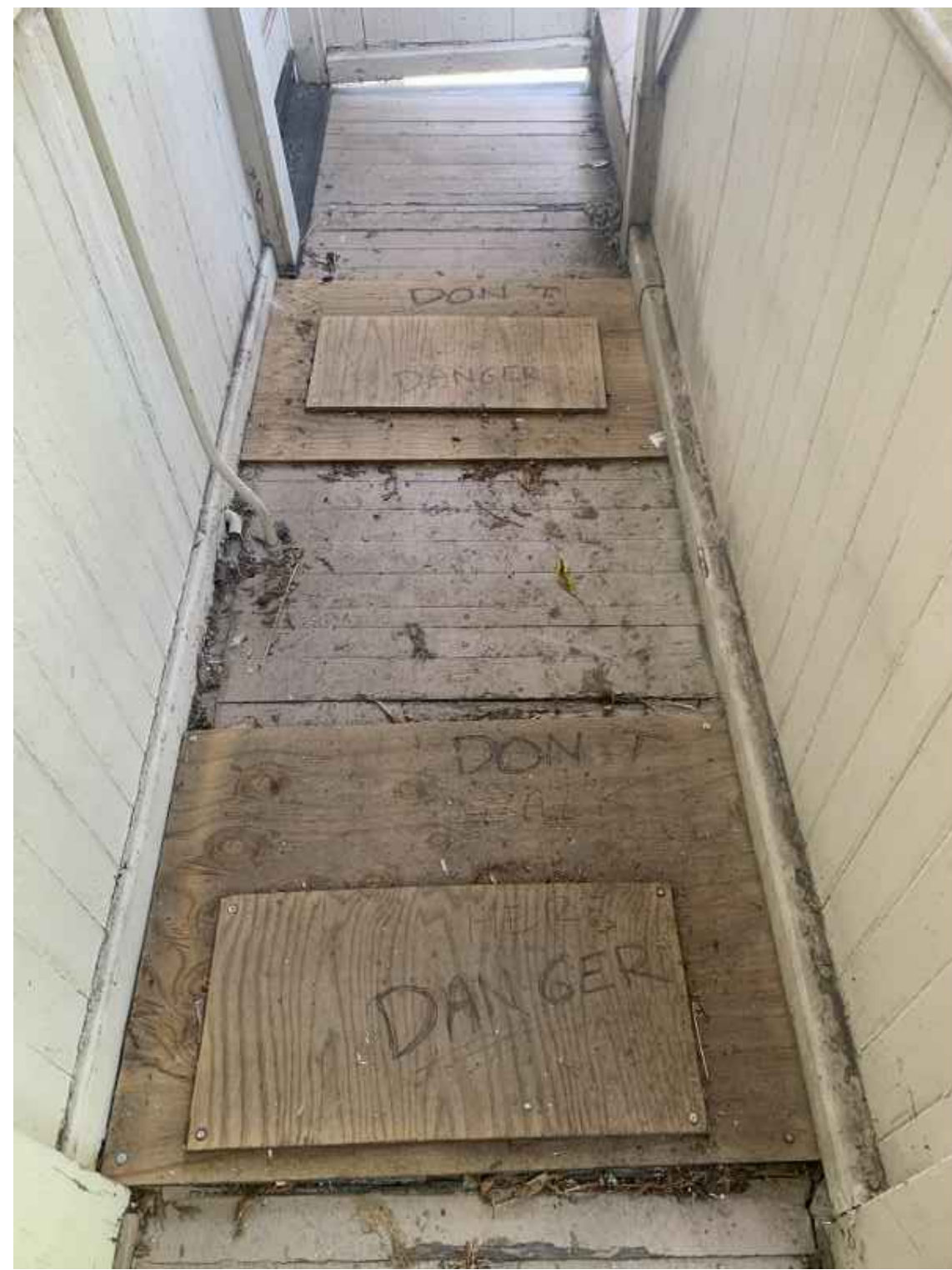
6 TYPICAL DAMAGED SLOPING LANDING
