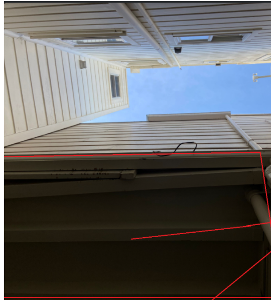
Exterior View: Third and partial Second Floors
