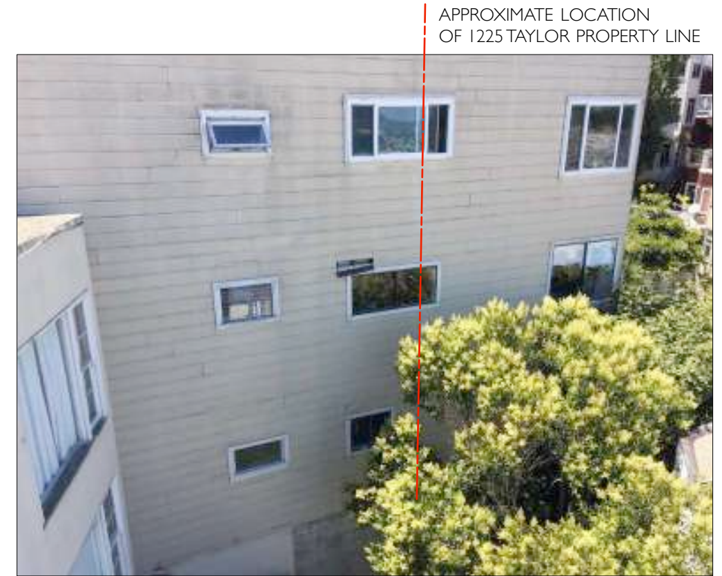
Recent photograph of rear portion of east elevation
