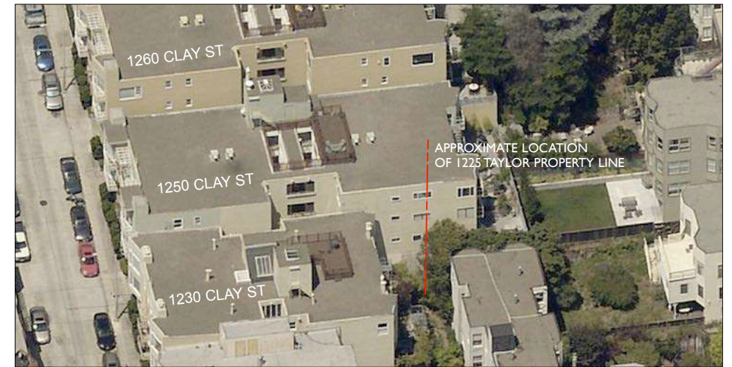
2014 aerial photograph of east elevations of 1230-1260 Clay Street buildings
