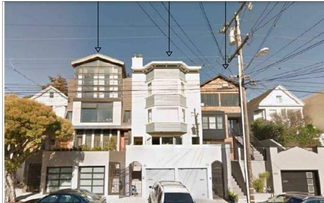
4 BUILDINGS ON THE OPPOSITE SIDE OF THE STREET A1.01 NTS
