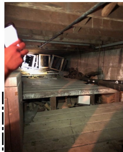
VIEW OF EXISTING BASEMENT TOWARD MISSION
