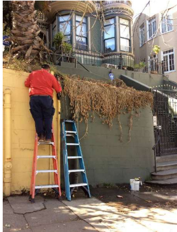
Photo 6 – Plumber repairing the water pipe.
