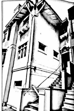
2 EXTERIOR FRONT PHOTOGRAPH (SOUTH) NTS 1550-1552 LAKE ST
