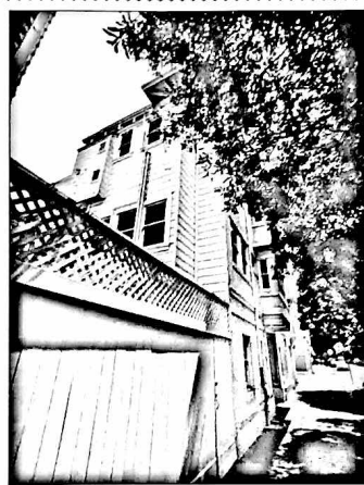
3 EXTERIOR REAR PHOTOGRAPH (NORTH) NTS 1550-1552 LAKE ST
