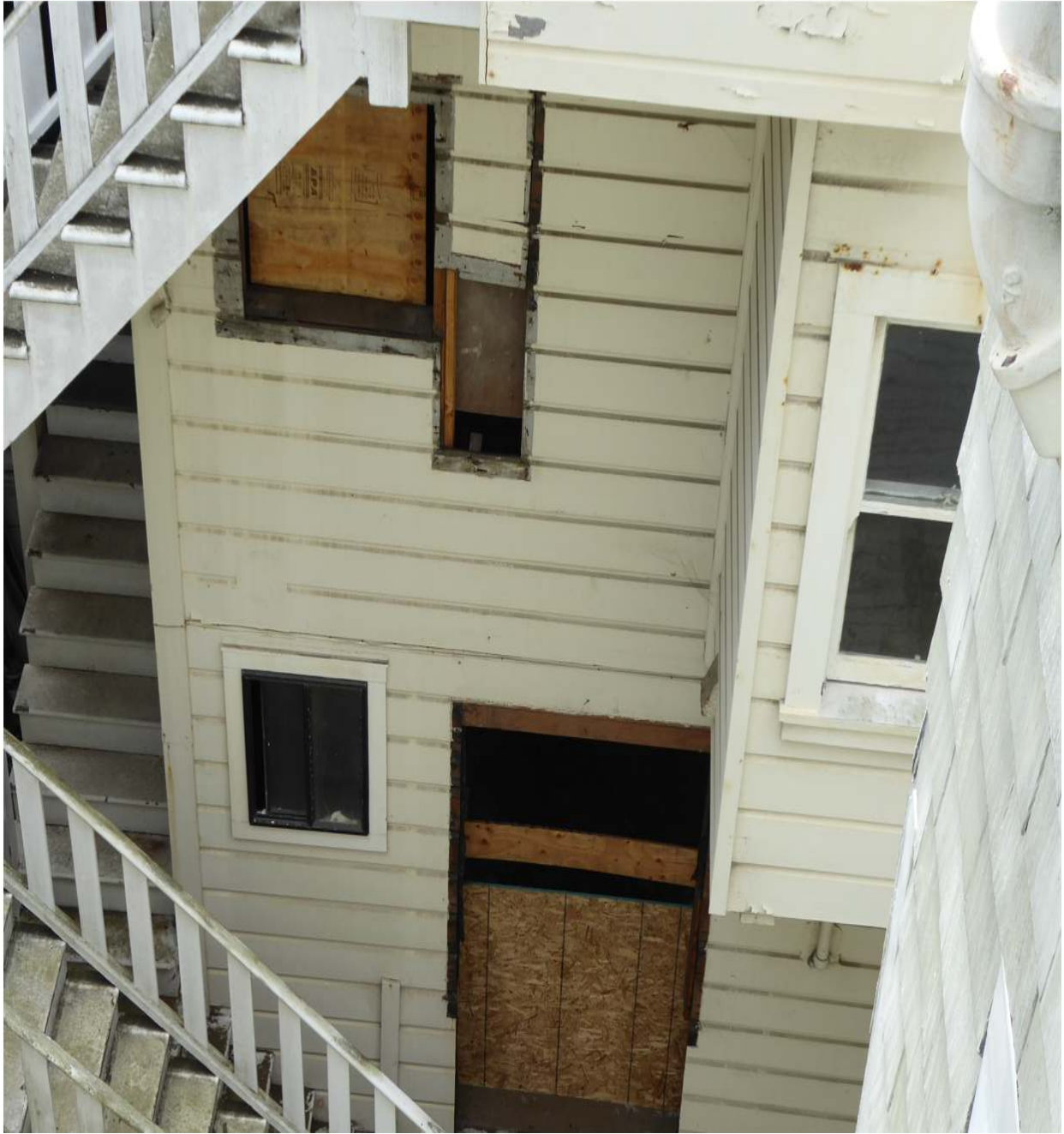
Three former North wall windows west of the former kitchen window
