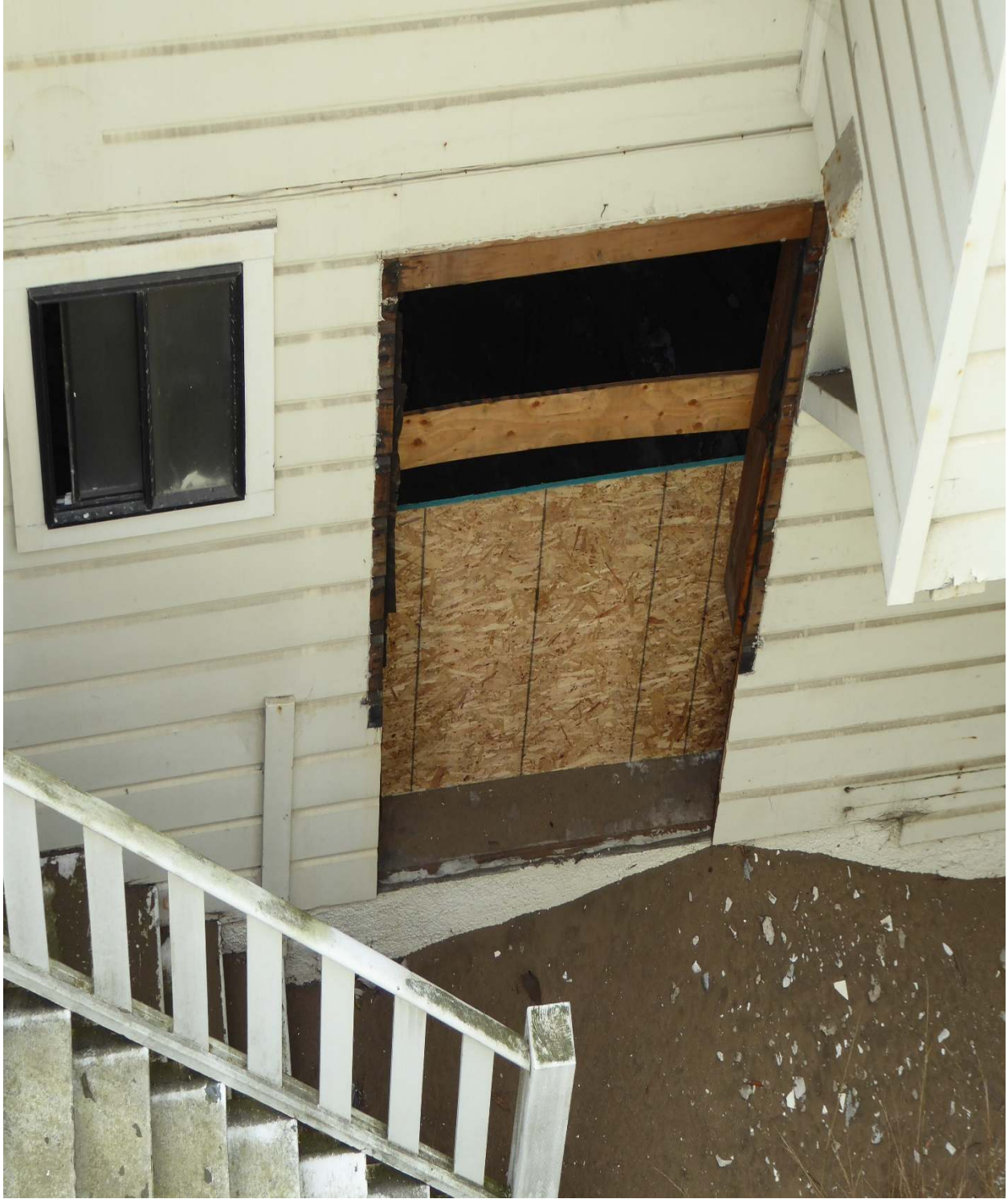
North wall ground floor window removed and opening expanded to doorway
