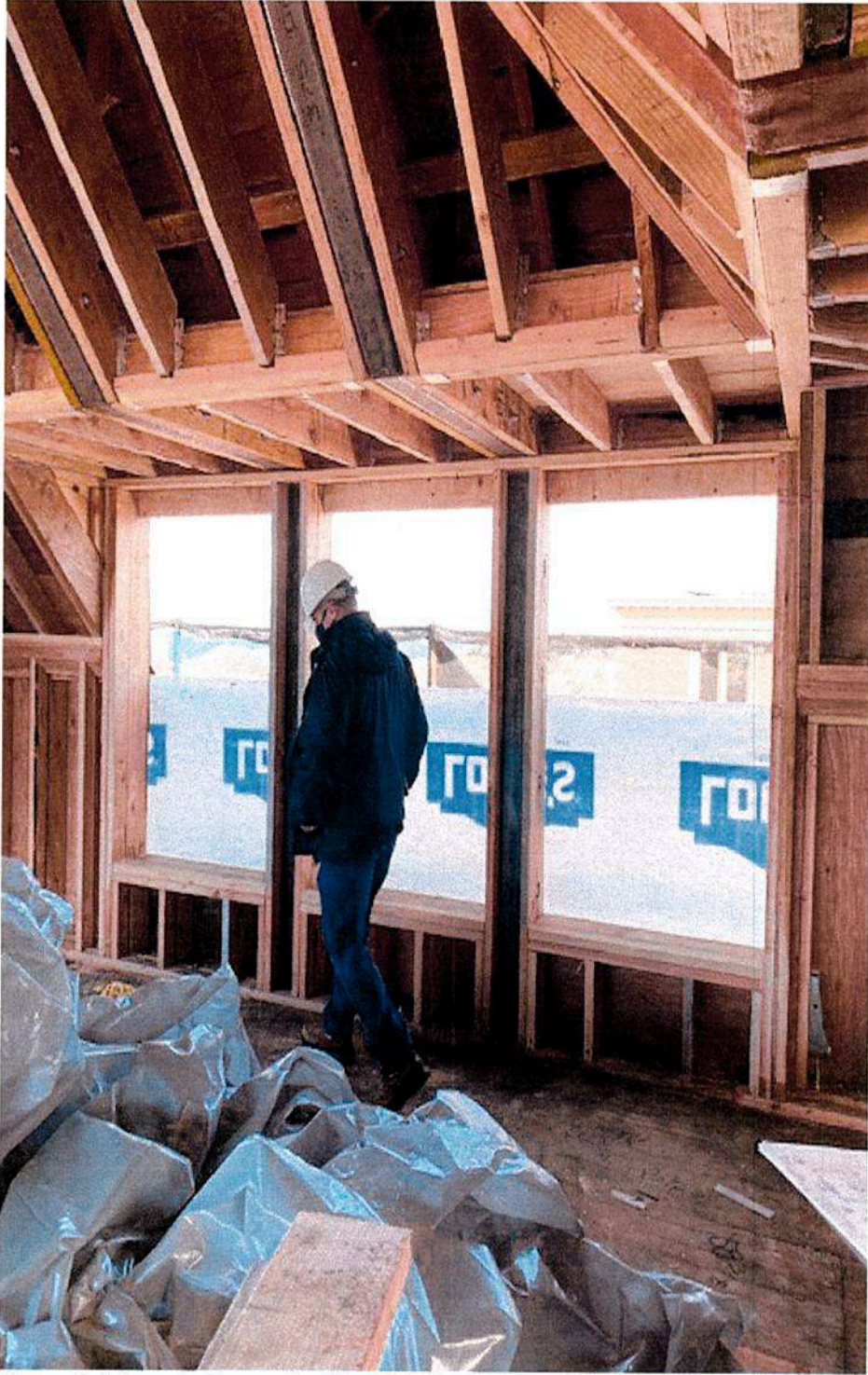
Figure 3 (above) shows the Fourth Floor Front Windows |
