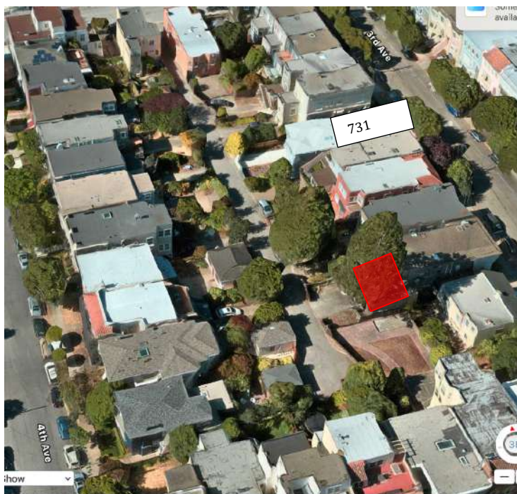
Figure 7. Aerial view of Block 1646 mid-block open space (facing North-East from Fulton ). This shows that the western extent of 731 3rd Avenue. The applicant has noted that there are other houses on 3rd Avenue that have reduced the mid block open space including 731 3rd Avenue. However, this is a far smaller house and the extension is not as large as one proposed for 757 3rd Avenue. Also seen is how house 765 would be boxed in by the extension.
