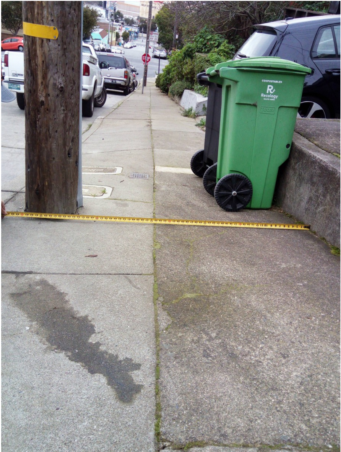
Sidewalk Measurement Confirming ADA Compliance
