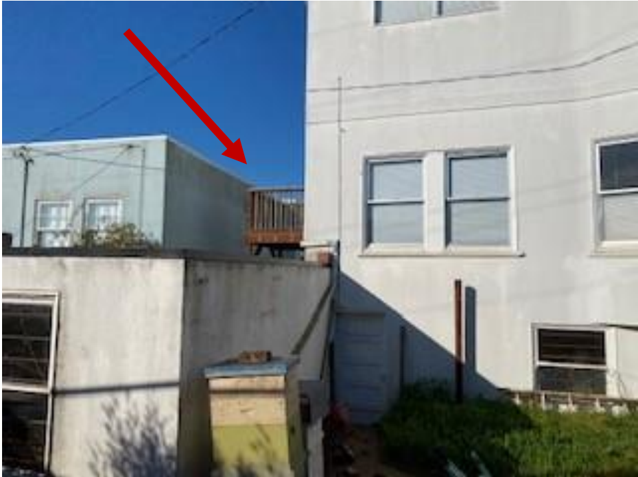
View from fence line 1417 Plymouth
