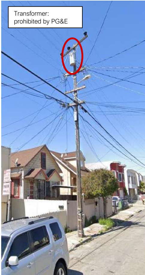
Figure 6: Transformer, Triangular Construction, Cutout
