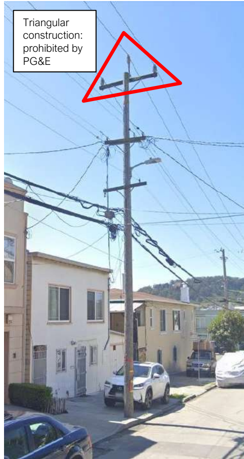
Figure 6: Transformer, Triangular Construction, Cutout
