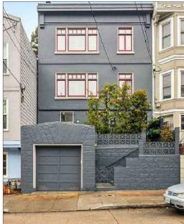
1 FRONT FACADE OF THE SUBJECT BUILDING A1.01 NTS
