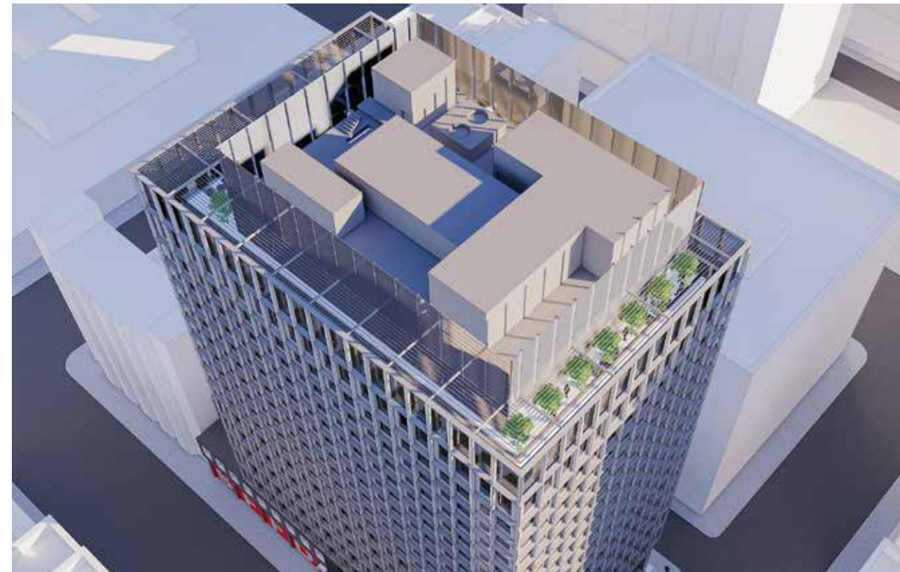
Crown Aerial View showing Roof Mech. Screen
