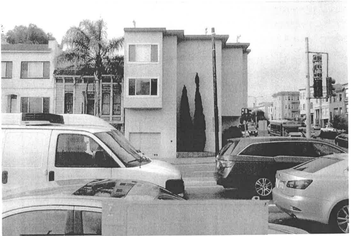
Looking south across Cesar Chavez Street from the proposed site. Guerrero is on the right, to the west.
