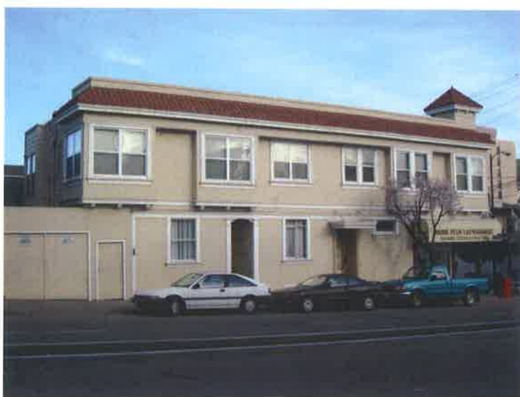
View looking southeast at the west façade. Source: San Francisco Planning Department
