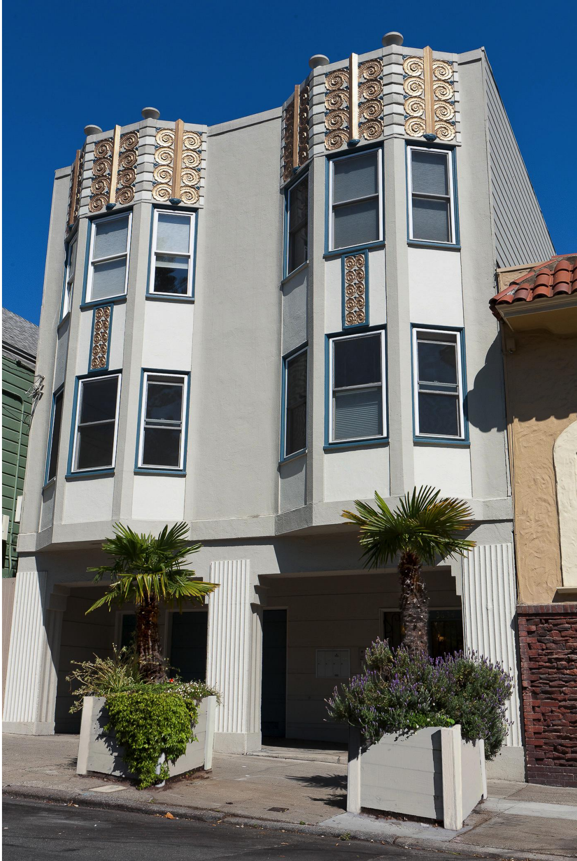
Photo Illustrating if Planter Boxes are Repaired & Painted to Match the Building
