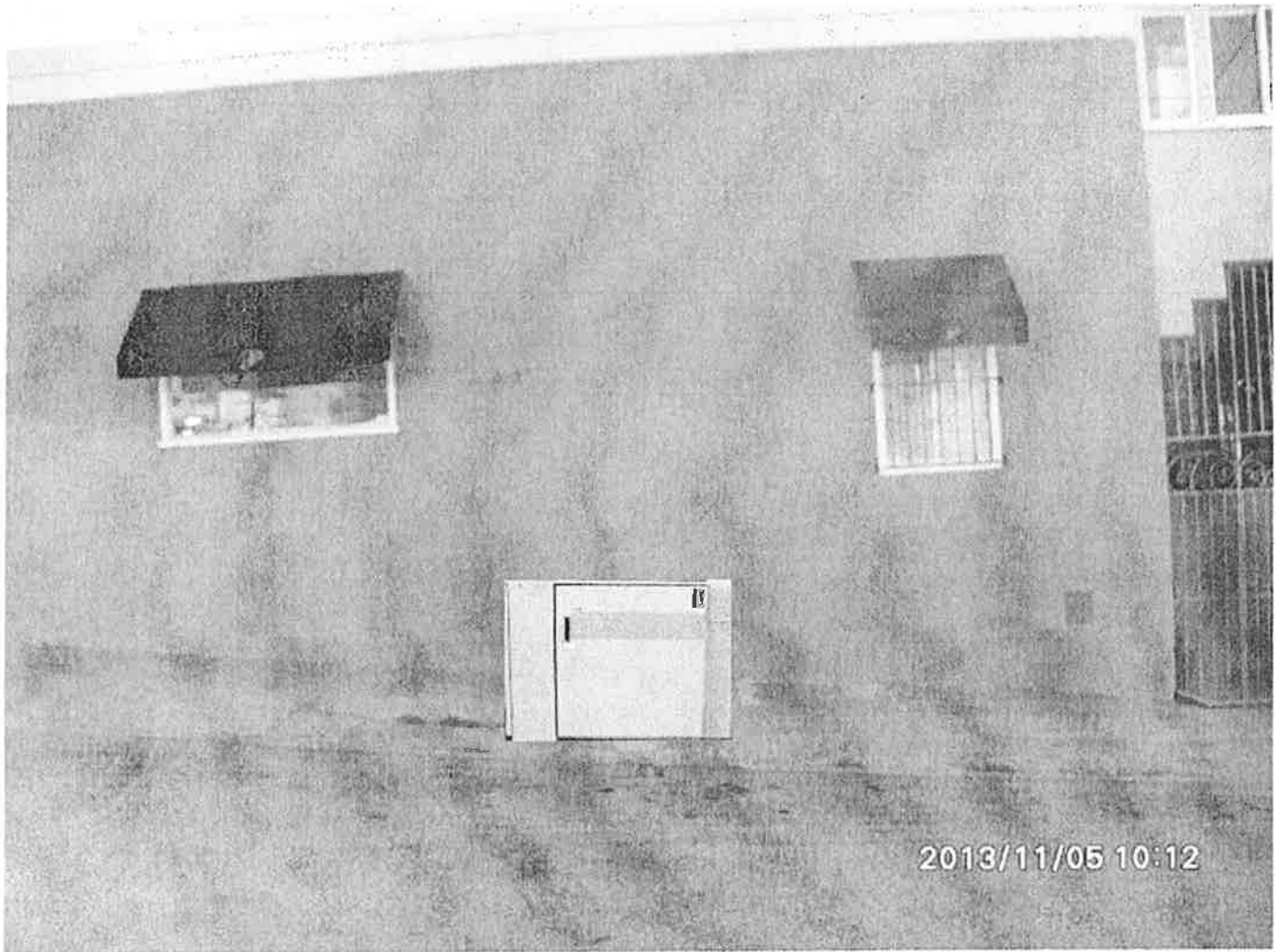
Looking east across Missouri Street, toward the proposed location 20 th Street is on the left, to the north
