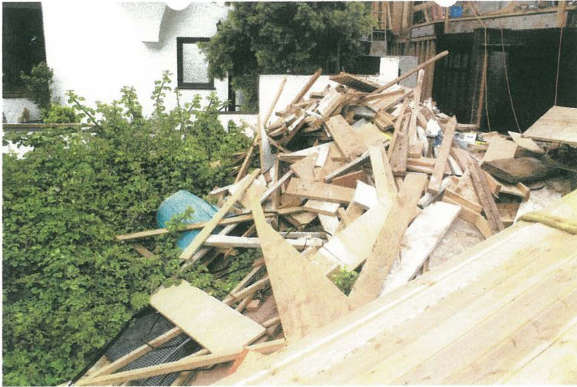
View Looking Back at Matula Home During Construction
