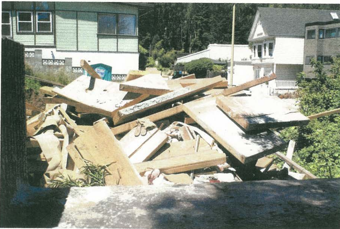
View From MATULA Home Looking West Across Stairs
