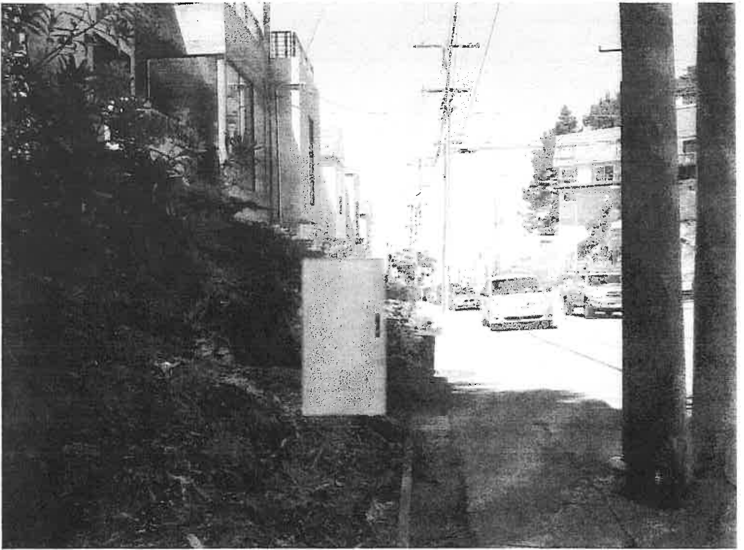
Looking west along the south sidewalk of Quintara St, toward 12 th Avenue.
