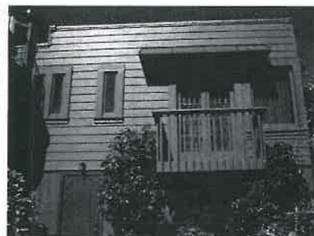
B: SUBJECT PROPERTY: SIDE VIEW
