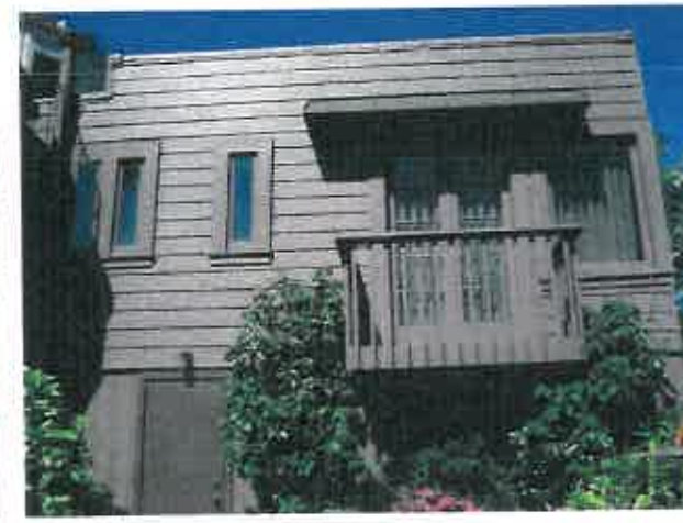
B: SUBJECT PROPERTY: SIDE VIEW
