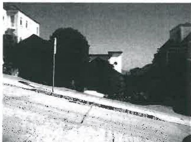
G: SUBJECT PROPERTY - STREET VIEW: 3660 21ST STREET
