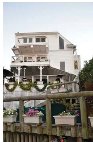
D: ADJACENT PROPERTY TO EAST - REAR VIEW: 3650 21ST STREET
