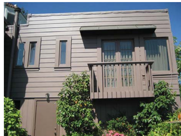
B: SUBJECT PROPERTY: SIDE VIEW
