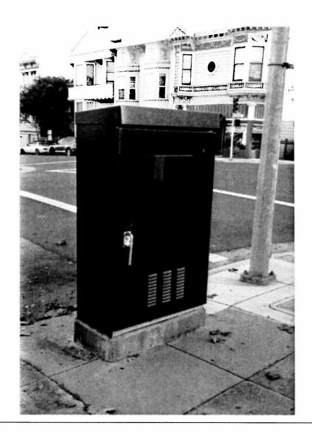
M-SF CONTROLLER CABINET: 36" W x 17" D x 60" H CONCRETE FOUNDATION: 38" W x 19" D x 6" H (portion above ground)
