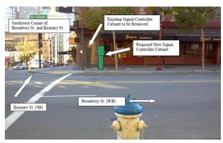
Upper controller cabinet is 24.25"W x 40"H x 17.5"D Lower pedestal cabinet is 20" W x 30"H x 16"D Pedestal cabinet base 17"W x 3"H x 13" D Concrete foundation is 17"W x 2"H x 13"D Total Height (cabinet & foundation): 75"
