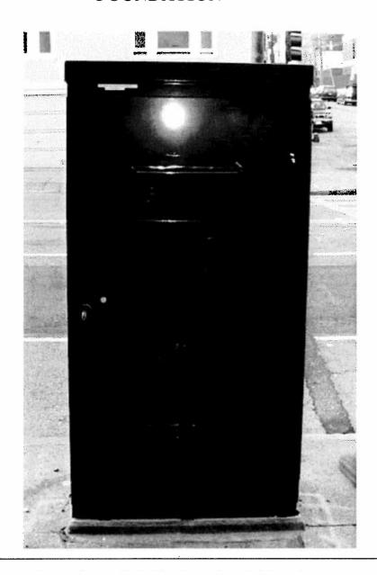
M-SF CONTROLLER CABINET: 36" W x 17" D x 60" H CONCRETE FOUNDATION: 38" W x 19" D x 6" H (portion above ground)
