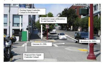
Controller cabinet is 36"W x 60"H x 17"D; Concrete foundation is 38"W x 6"H x 19"D Total Height (cabinet & foundation): 66"
