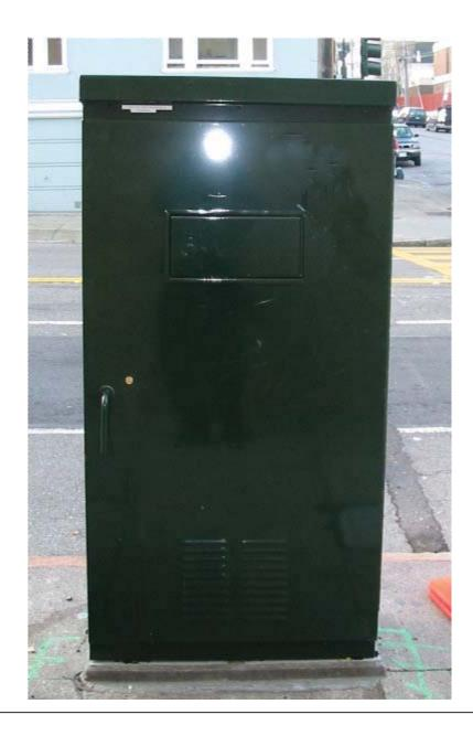
M-SF CONTROLLER CABINET: 36" W x 17" D x 60" H CONCRETE FOUNDATION: 38" W x 19" D x 6" H (portion above ground)
