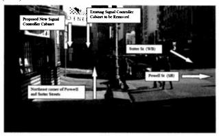
Upper controller cabinet is 24.25"W x 40"H x 17.5"D Lower pedestal cabinet is 20" W x 30"H x 16"D Pedestal cabinet base 17"W x 3"H x 13" D Concrete foundation is 17"W x 2"H x 13"D Total Height (cabinet & foundation): 75
