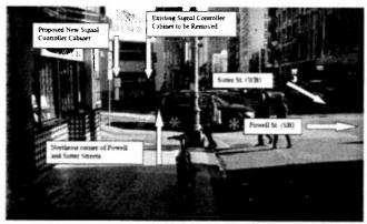
Upper controller cabinet is 24.25"W x 40"H x 17.5"D Lower pedestal cabinet is 20" W x 30"H x 16"D Pedestal cabinet base 17"W x 3"H x 13" D Concrete foundation is 17"W x 2"H x 13"D Total Height (cabinet & foundation): 75 Division of Sustainable Streets - Transportation Engineering Municipal Transportation Agency One South Van Ness Avenue, 7<sup>th</sup> Floor San Francisco, CA 94103-5417
