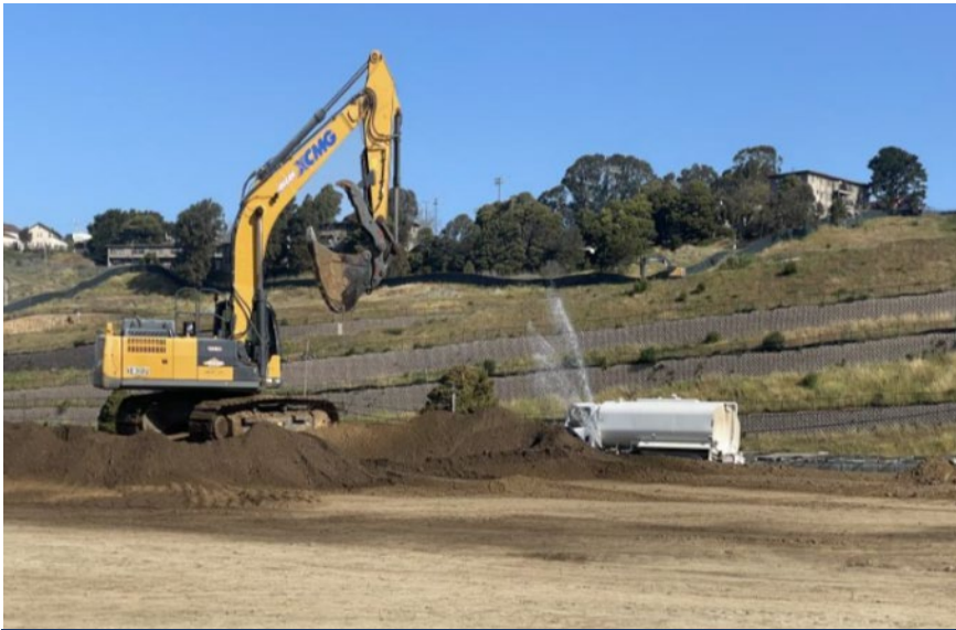
Dust is managed during installation of clean fill
