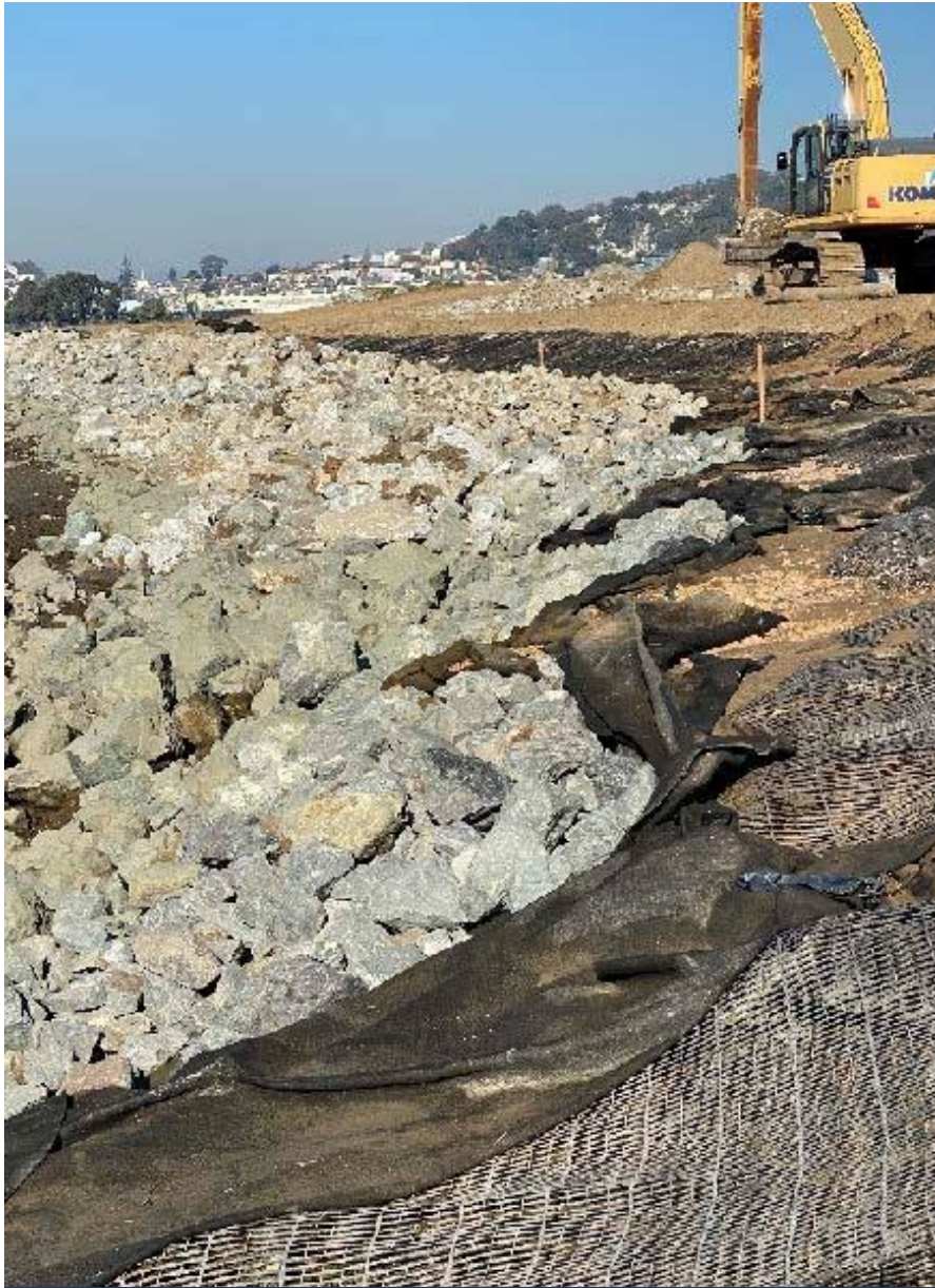
Installation of filter stone and rip rap
