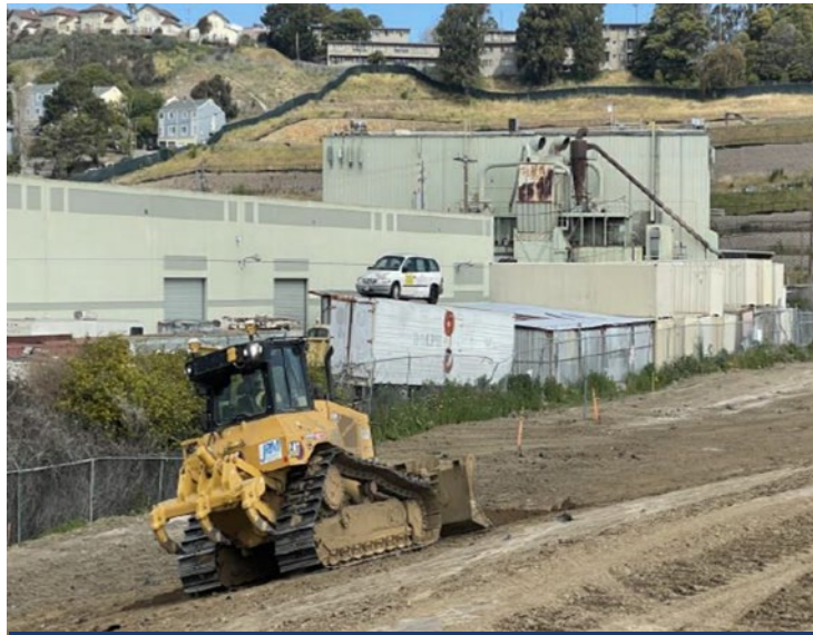
Site grading and compaction is ongoing
