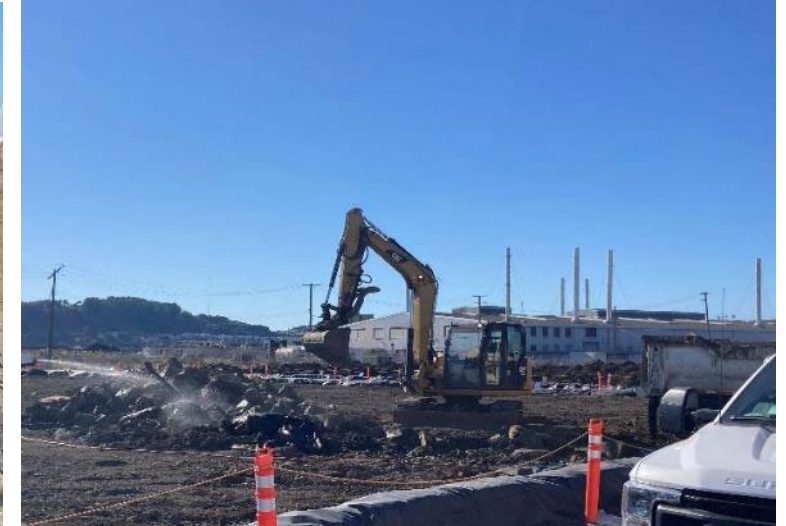
Dust management on radiological screening yard (RSY) pads at IR-03
