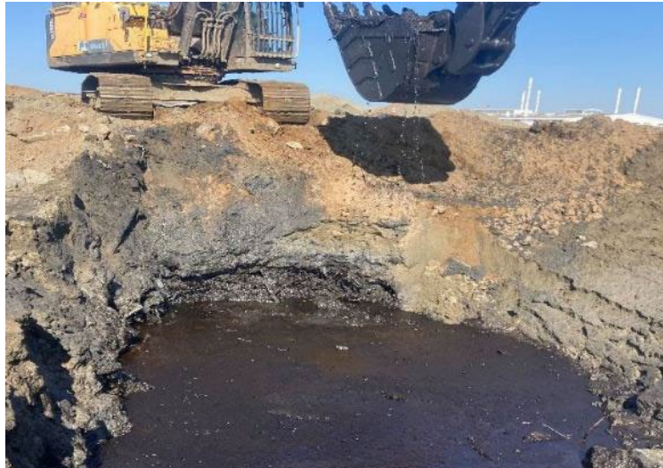
Close-up of excavated area at IR-03 shoreline (Grid #8)
