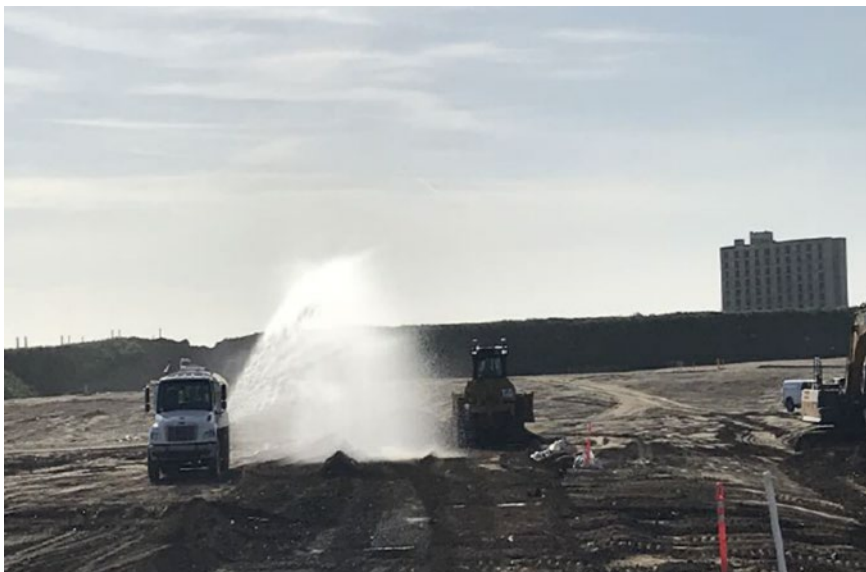
Dust is controlled during site grading
