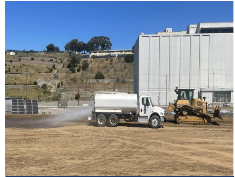
Dust is managed during site work
