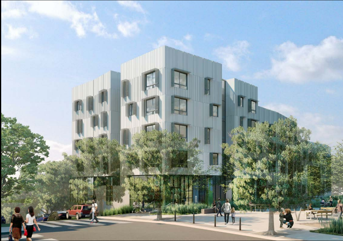
Block 14 southwest corner at Hunters View Drive – looking northeast
