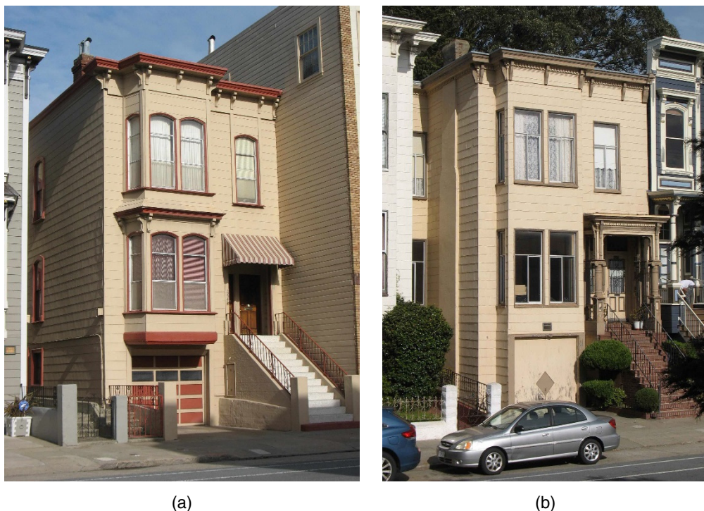
Figure 2-6 Victorian rowhouses with perimeter masonry chimneys: (a) restrained within the exterior wall sheathing; (b) unrestrained.
