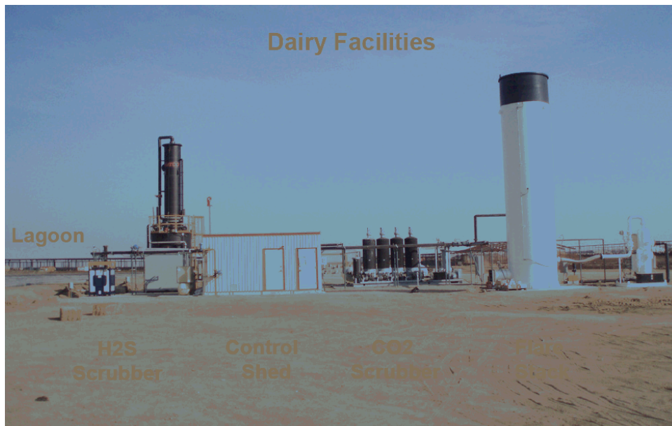
Figure 2. Clean-up System for Dairy Biogas prior to Injection in PG&E Pipeline
