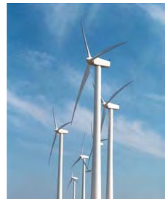
Figure 5-2 - Montezuma-3 Wind Turbines
