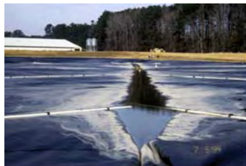
Figure 7-1 - Covered Lagoon Digester
