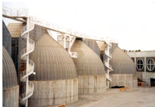
Figure 7-3 - Upright Mix Digesters
