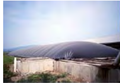
Figure 7-2 - Plug Flow Digester
