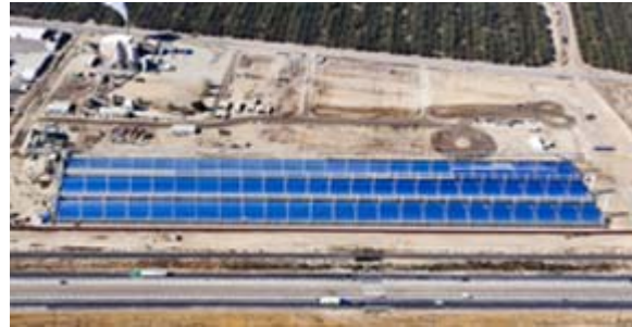
Figure 4-3 - Solar Thermal Installation
