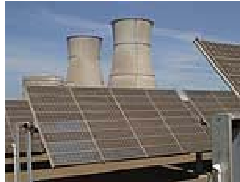
Figure 4-2 - Ground-Mounted PV System
