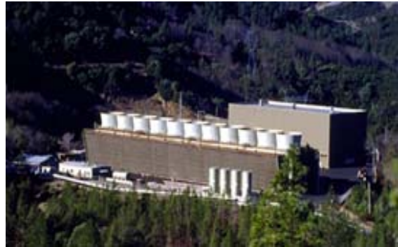
Figure 4-13 - Geothermal Power Plant
