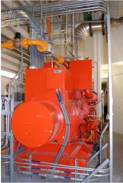
St. Mary's 750kW cogeneration system, providing heat, power, and savings.
