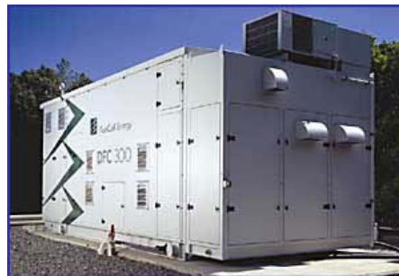
Figure 9: A 250kW FuelCell Energy fuel cell installed at a business [9].
