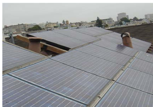
Figure 4-1 - Roof-Mounted Solar System
