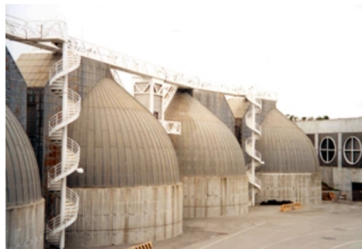
Figure 7-3 - Upright Mix Digesters
