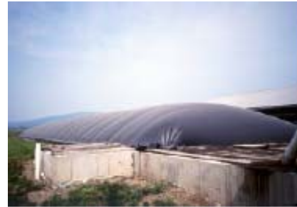
Figure 7-2 - Plug Flow Digester
