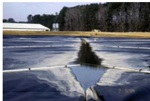
Figure 7-1 - Covered Lagoon Digester
