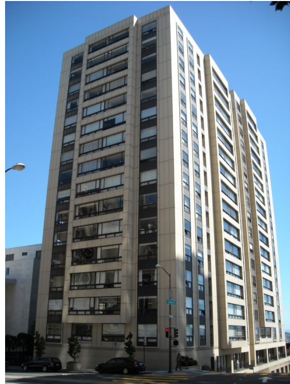
Figure 2. Modern Multifamily Property Year Built 1978 Hydronic heating used for space heating
