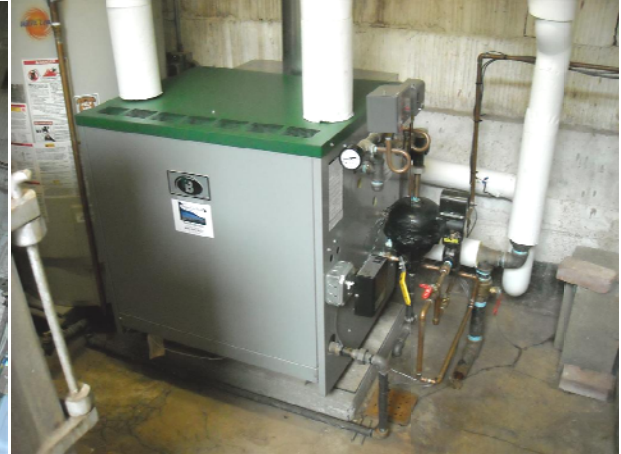
Figure 5. New low-pressure steam boiler (close up) New hot water heater in corner
