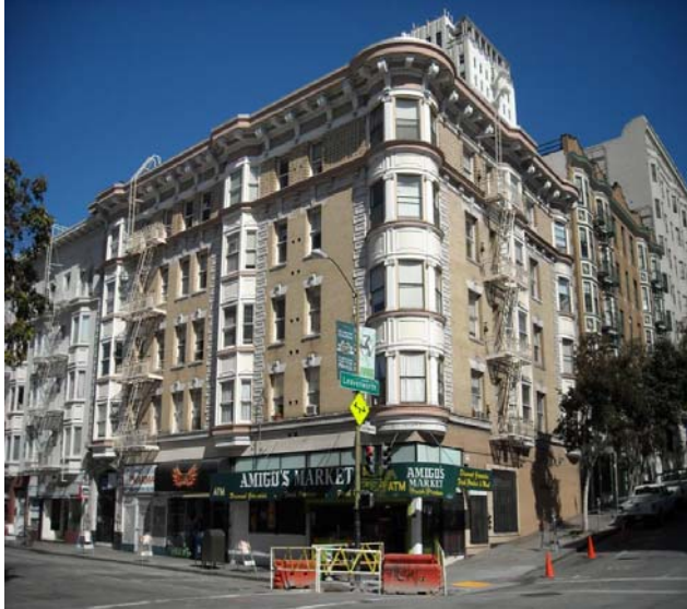
Figure 1. Prewar Era Multifamily Property Year Built 1910 Low-pressure steam used for space heating
