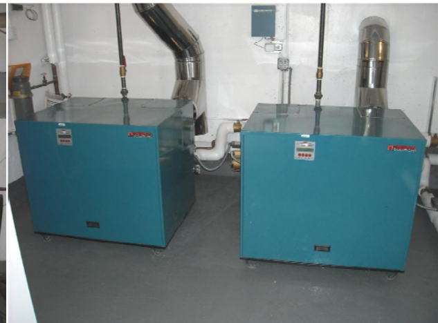
Figure 7. New High Efficiency Water Heaters
