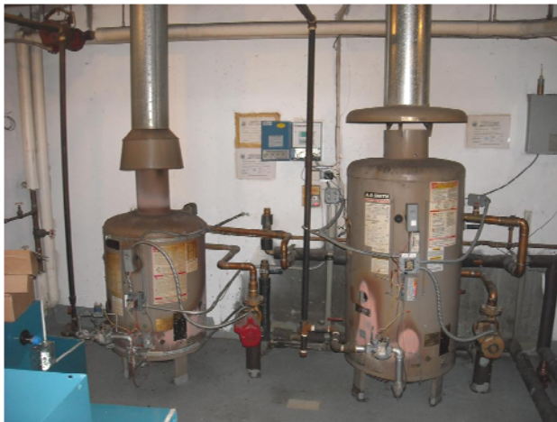
Figure 6. Existing Water Heaters
