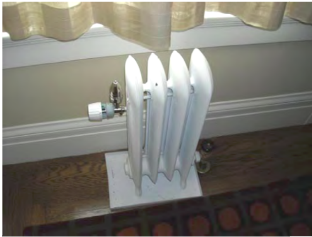
Figure 8. One-pipe low-pressure steam Thermostatic Radiator Valve (TRV)
