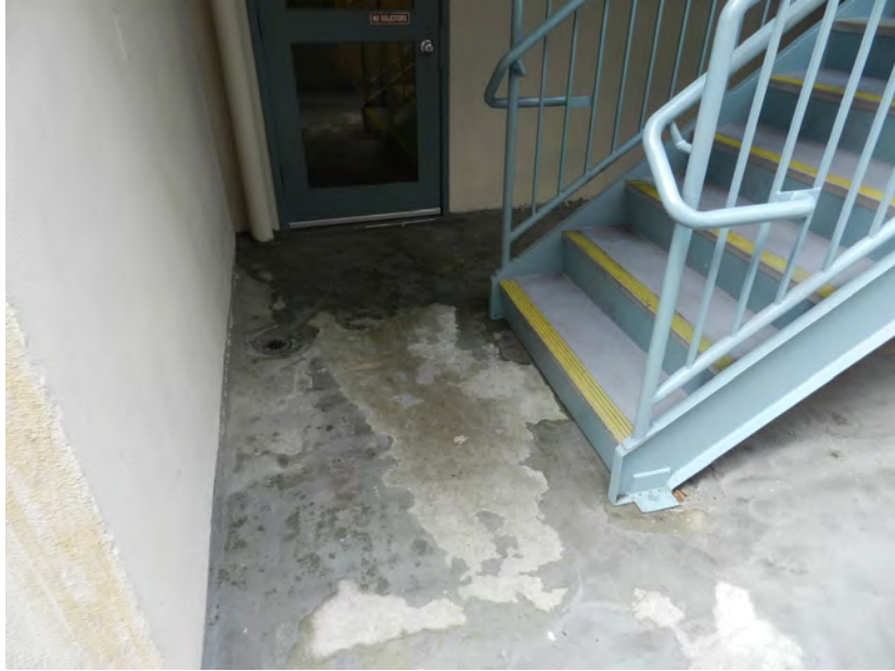
Stair at level 1 with corridor entry door beyond
