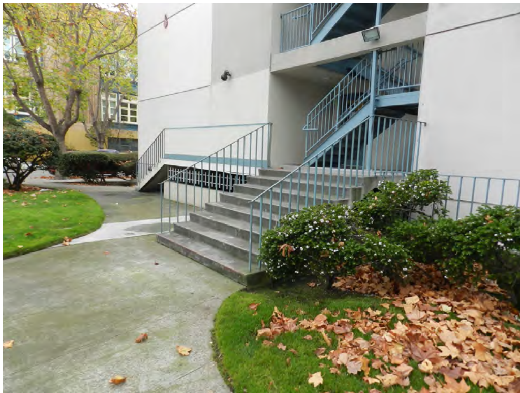
1415 Scott – north side steps and access stairs
