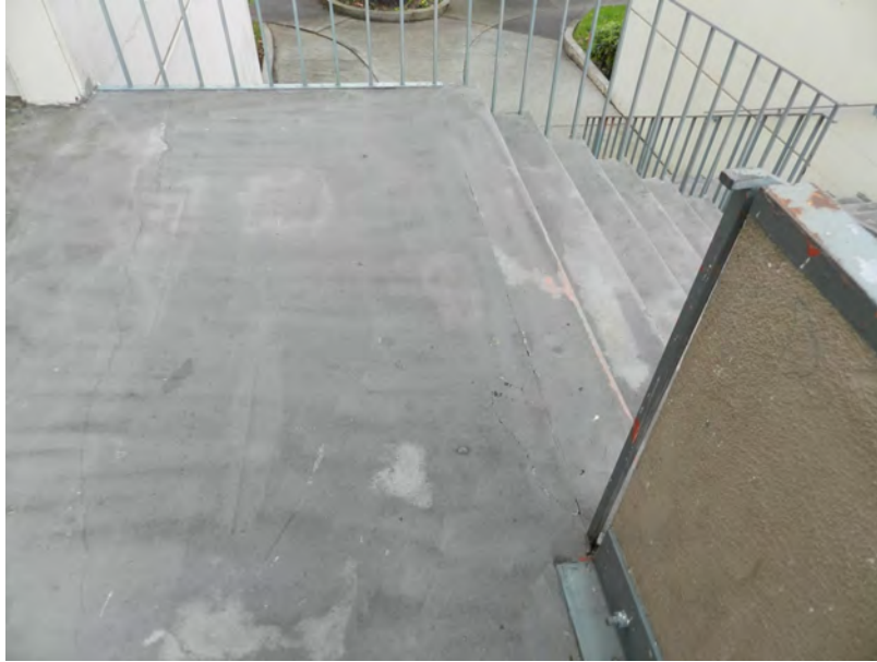
Landing at approach stairs at 2060 O'Farrell
