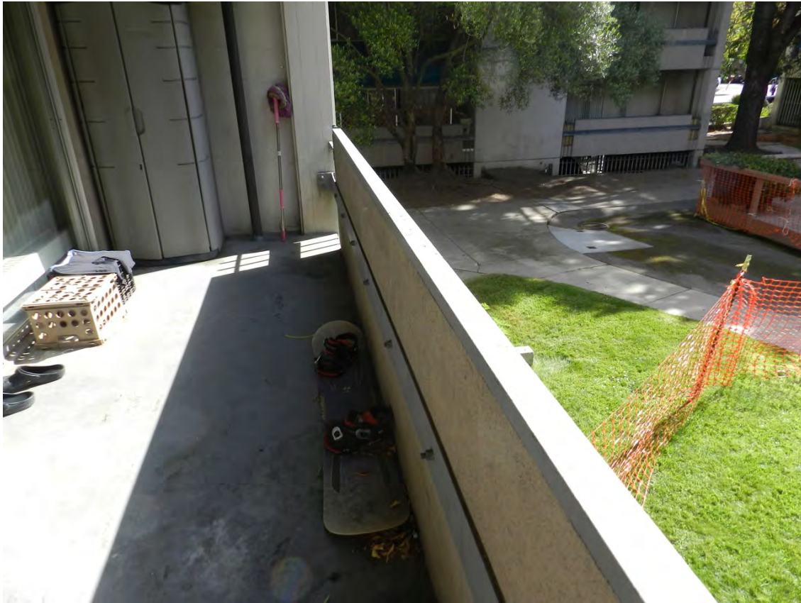
Balcony – Solid wall and deck surface
