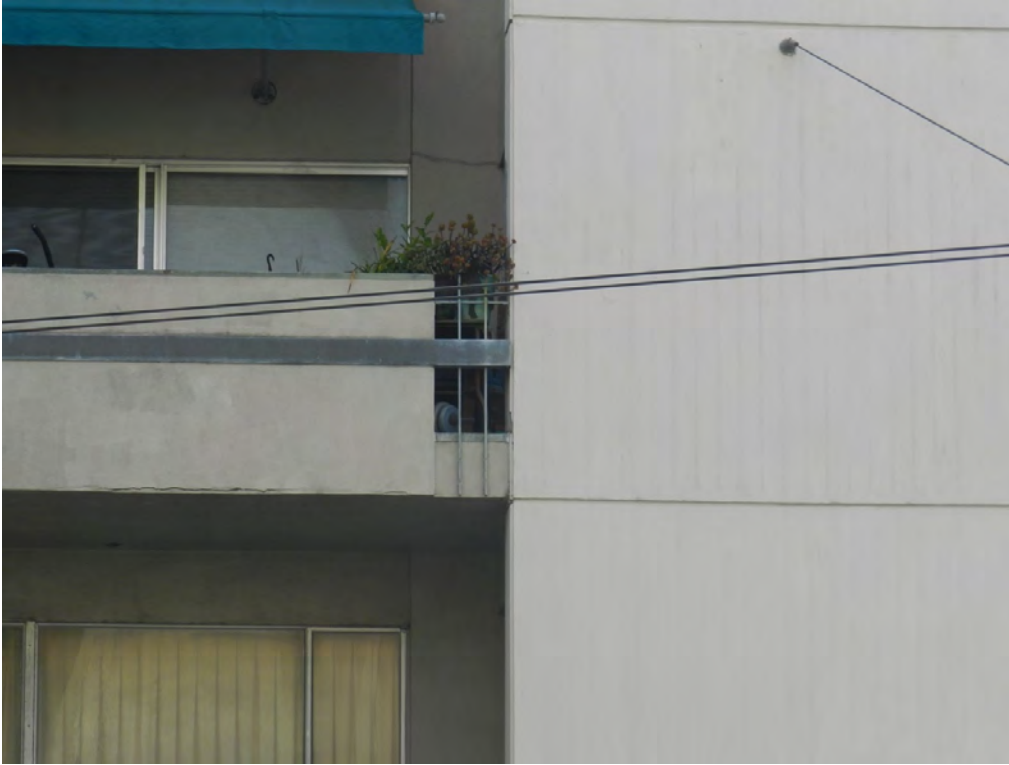
Building Exterior of 1450 Divisadero
