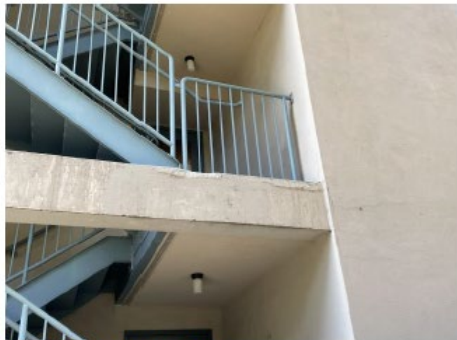
TYPICAL BEAM SPALLING
