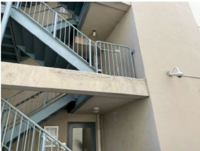
TYPICAL BEAM SPALLING
