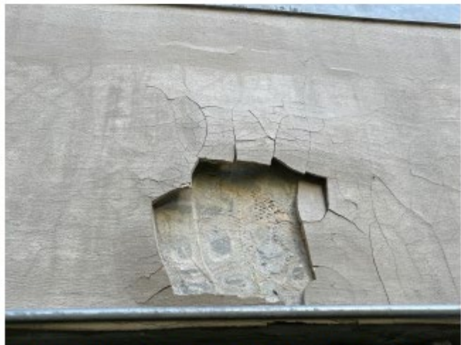
TYPICAL BALCONY GUARDRAIL DETERIORATION
