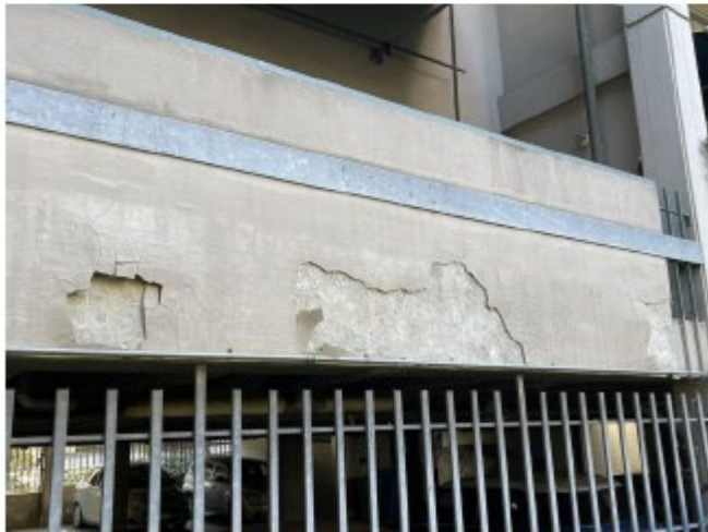
TYPICAL BALCONY GUARDRAIL DETERIORATION
