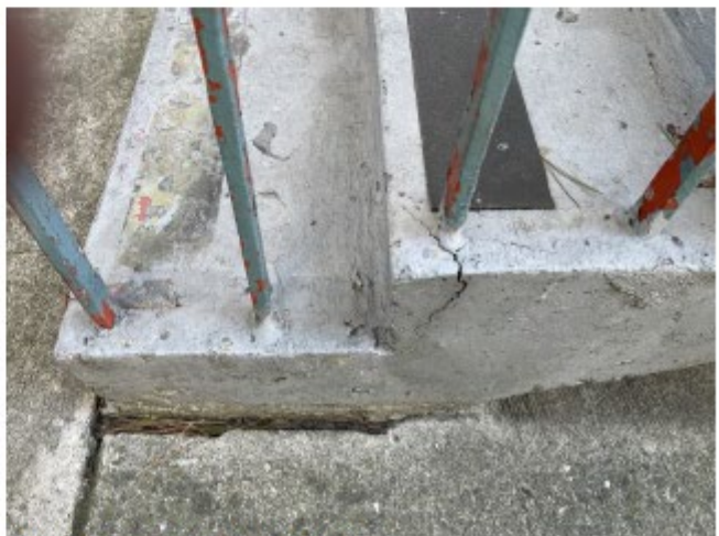
STAIR RAIL PICKET SPALLING
