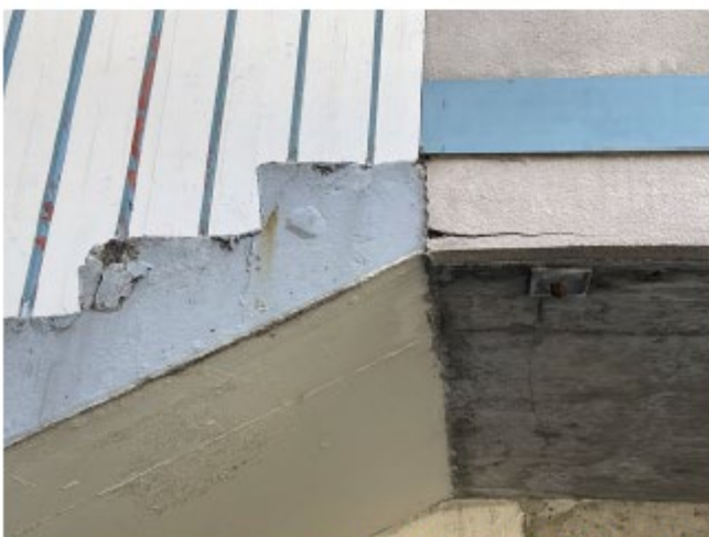
STAIR RAIL PICKET SPALLING
