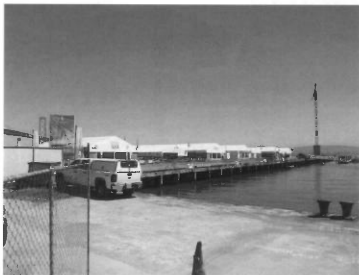
Subject Piers 30 and 32 view northeast
