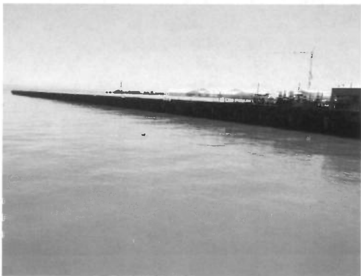
Subject Piers 30 and 32 view south
