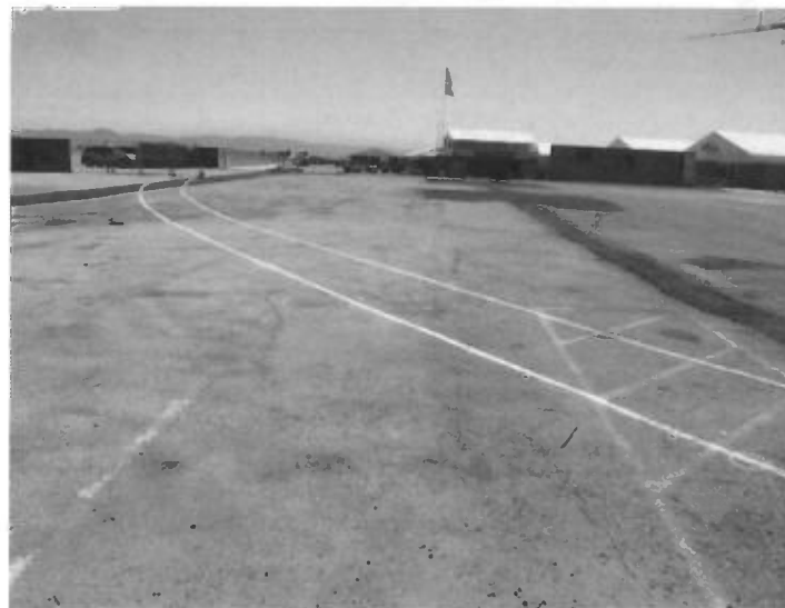
Subject Piers 30 and 32 view east
