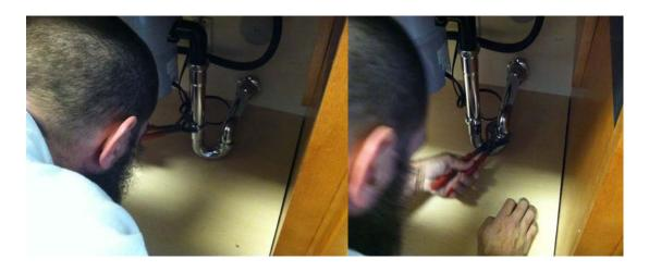
Using a wrench, remove the compression nuts (2 each) which connect the pea trap to the drain line of the sink, as shown above. There is (1) compression nut on each side of the pea trap elbow.
