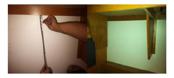
Re-attached ledger and support bracket at new location which was marked in step 1.
