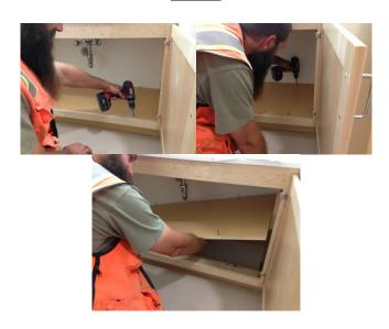
Remove the vanity base by removing (1) screw from each corner as shown above.
