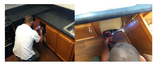
Remove screws from the cabinet frame located at the far left cabinet door and far right cabinet door (below the sink). There is (1) screw above and (1) screw below the cabinet door hinges, for a total of 4 screws, (2) on the left door and (2) on the right door.
