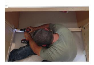
Remove the lower rail by removing (2) screws, (1) on either side, as shown above.
