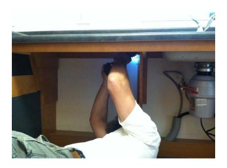
Remove the screws that attach the ledger to the back and sides of the countertop. The ledger is located under the countertop along the back wall and to the left & right sides of the countertop.
