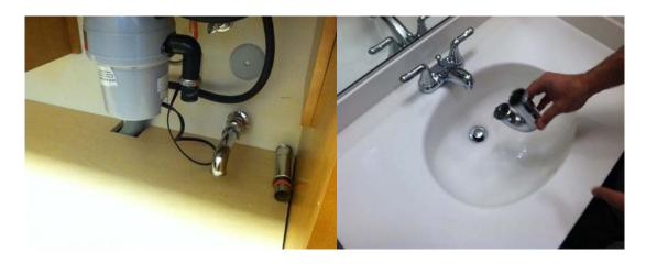
Once the pea trap is removed, the waste line assembly should look like the above left photo.
