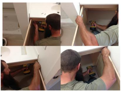
Remove the (2) doors by removing the (2) screws from each door, as shown above.
