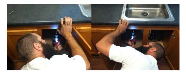
Remove the screws from the inside of the cabinet face at the top of the cabinet door opening as shown above.
