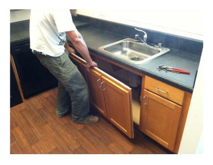
Remove Cabinet Face-Frame with the (4) cabinet doors attached.
