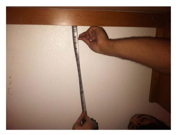
Measure 2" down from the bottom of the ledger and mark the new location on the wall; this will be the new location for the ledger once lowered.
