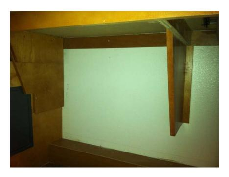
Remove the support bracket centered underneath the countertop.
