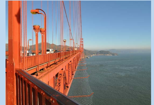
Golden Gate Bridge Suicide Deterrent Net System
