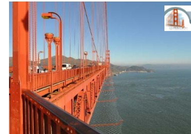
Golden Gate Bridge Suicide Deterrent Net System
