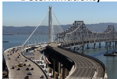
Bay Bridge Rebuild
