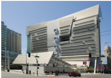
Federal Building at 7 th & Market
