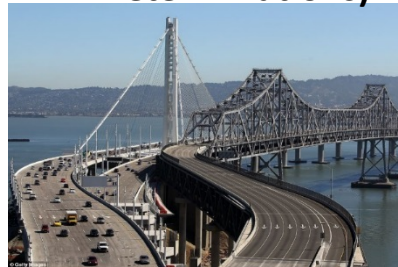
Bay Bridge Rebuild
