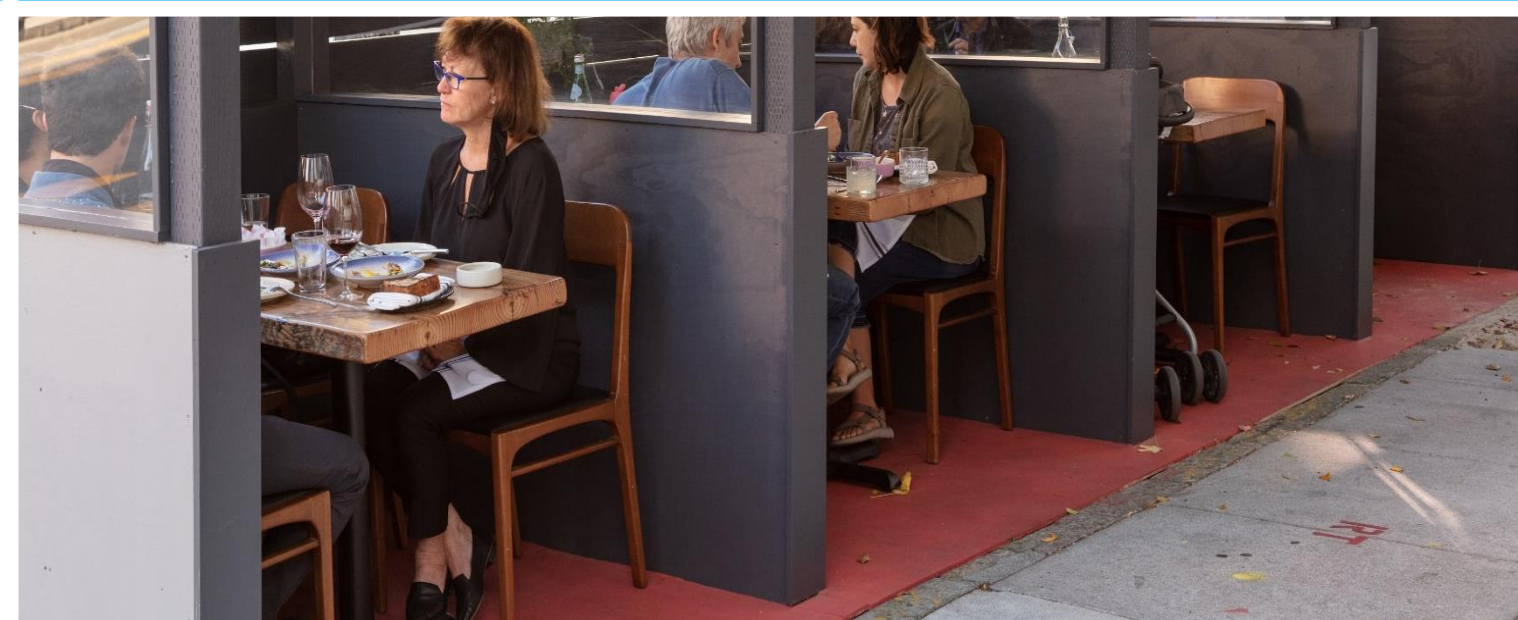
Deck Threshold Level With Sidewalk
