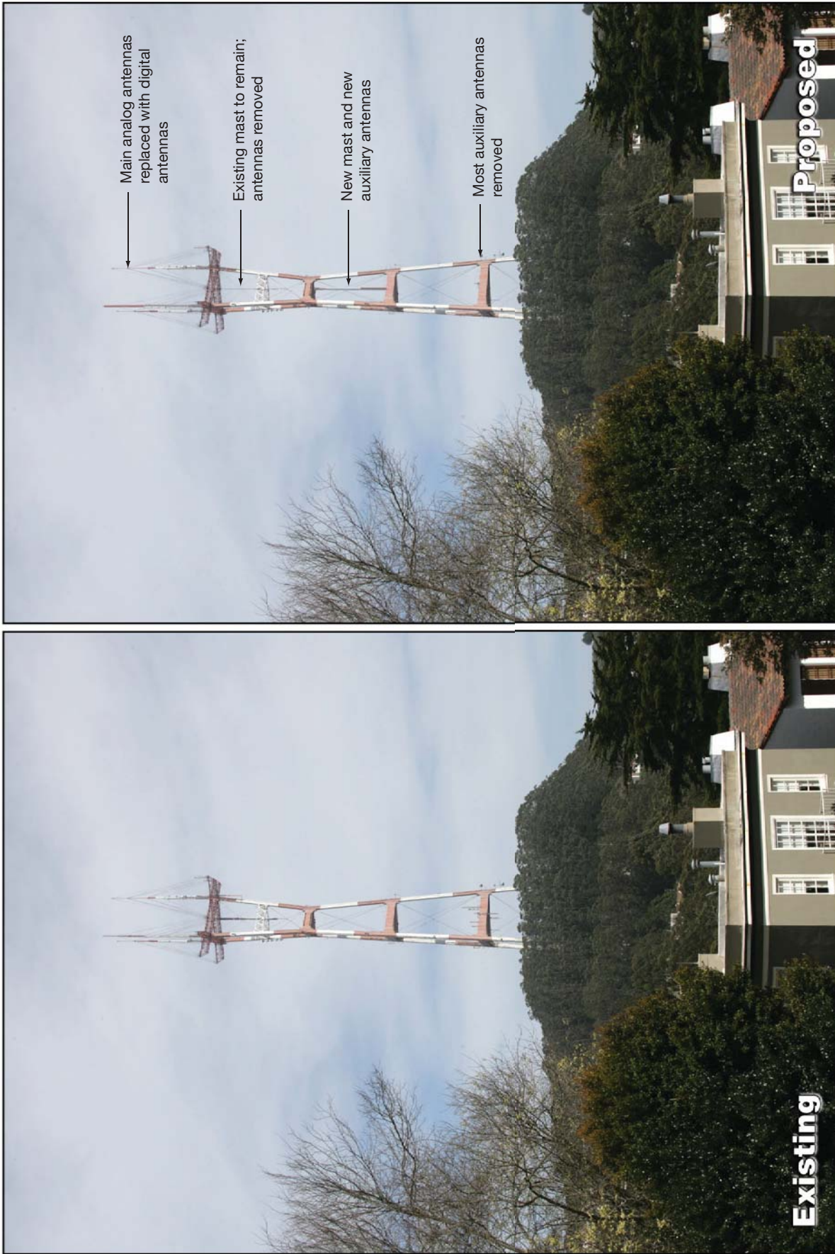
2007.0206E: Sutro Tower Digital Television - 2066334 Figure 7 Photosimulation of View Looking Northeast from 9th Avenue near Pacheco Avenue
