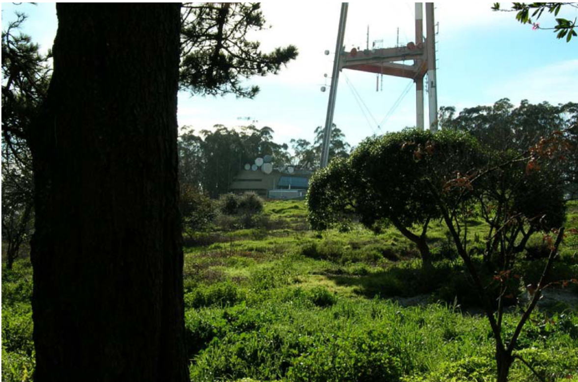
Base of Sutro Tower and Transmission Building seen from Marview Way near Farview Court
