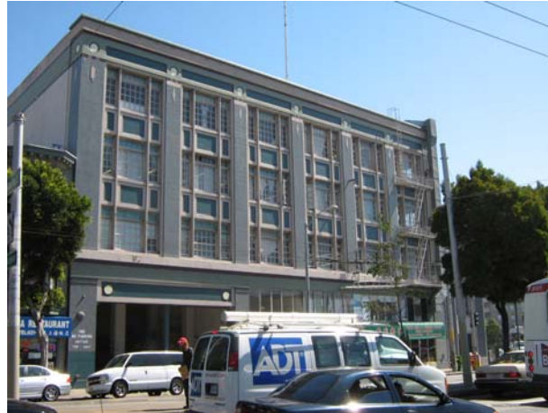
Figure 39: 1563 Mission Street, built 1917. Source: Page & Turnbull
