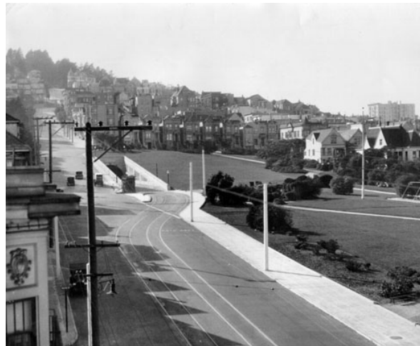
Figure 34. Duboce Park with Duboce Tunnel in background, 1929.
