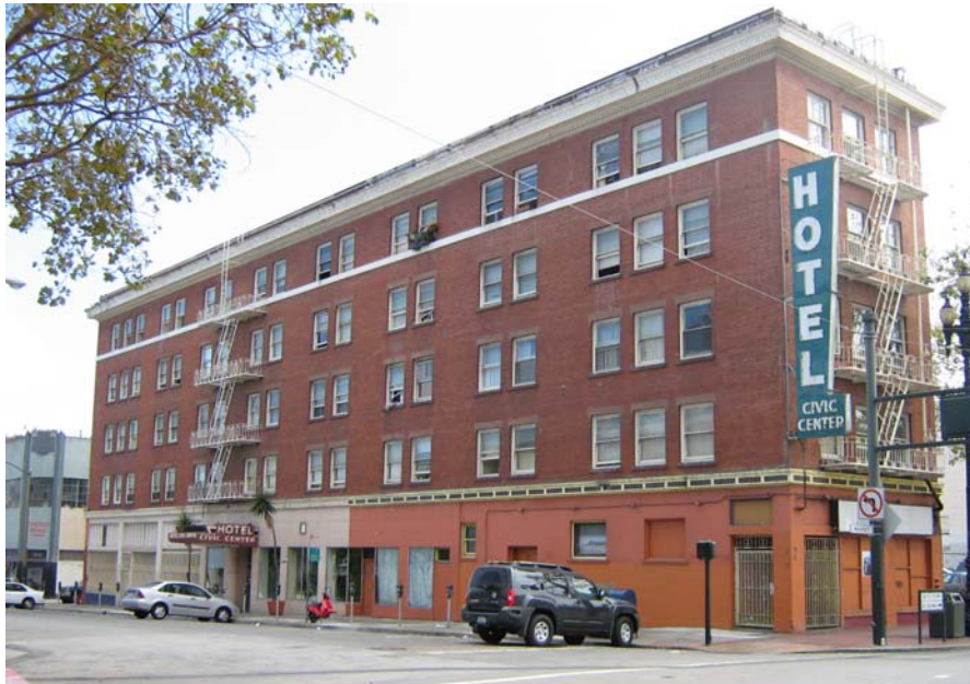
Figure 45. SRO at 1601 Market Street. Source: Page & Turnbull
