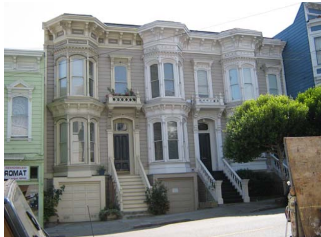
Figure 9. Rowhouses at 615-29 Hayes Street. Source: Page & Turnbull
