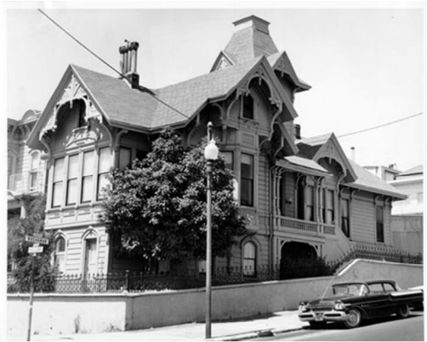
Figure 10. Nightingale House, 201 Buchanan Street. Source: San Francisco Public Library
