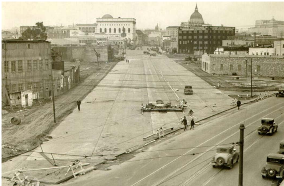
Figure 29. South Van Ness Avenue Extension, 1931. Source: San Francisco Public Library
