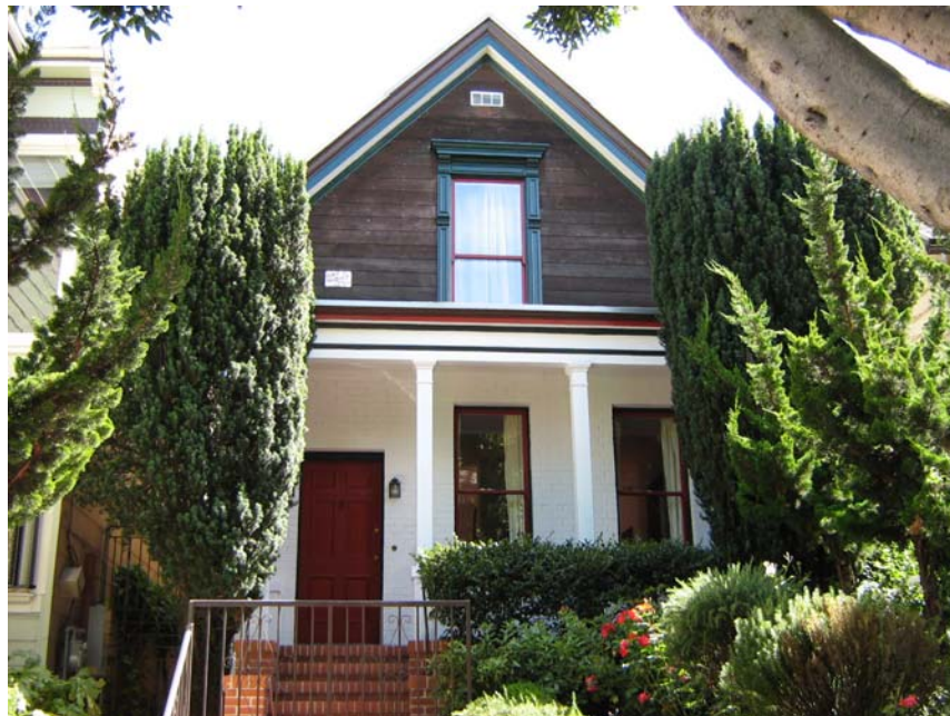
Figure 50. Single-family dwelling at 2173 15 th Street in Duboce Triangle, ca. 1875. Source: Page & Turnbull
