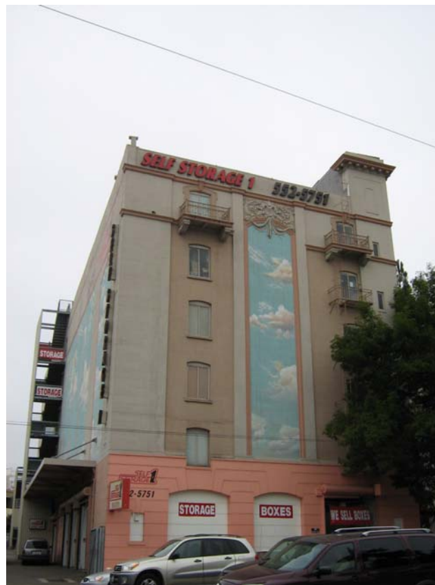
Figure 59. Bekins Warehouse, 190 Otis Street in the South of Market, built 1906 and reconstructed 1909. Source: Page & Turnbull
