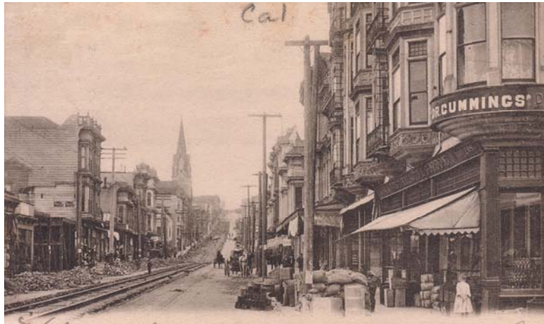
Figure 24. Earthquake damage along Hayes Street, 1906. Source: Collection of Glenn Koch
