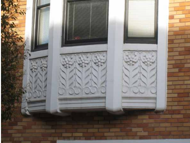
Detail of window bays. Source: San Francisco Planning Department
