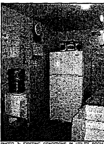
PHOTO 3: EXISTING CONDITIONS IN UTILITY ROOM.
