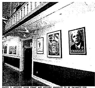
PHOTO 3: HISTORIC DOOR FRAME AND HISTORIC WANSKOT TO BE SALVAGED FOR REINSTALLATION.
