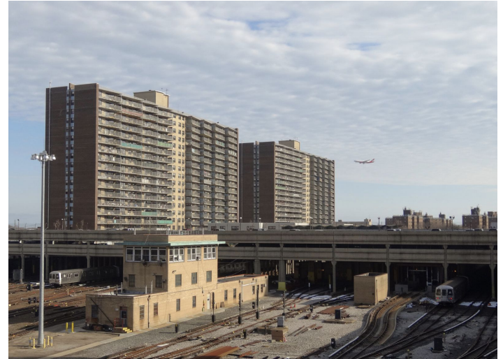
Pitkin Yard in New York City, housing development on a deck over active subway yard, 2 others like it in NYCT Subway System
